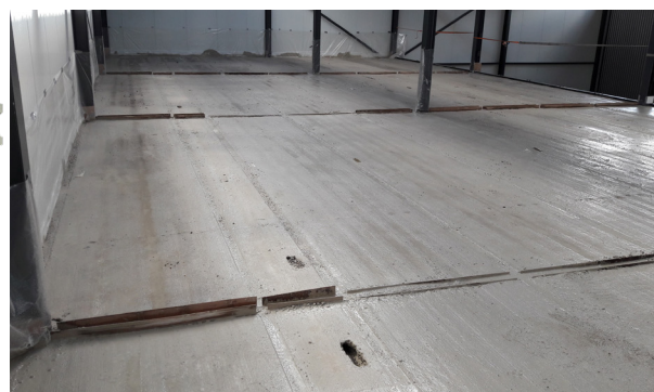
Fig. 7-13 Detail of hollow-core floor to beam joint in the middle of the building and the floor field where hollow-core slab ends are closed with thin plates detaching them from the beams
