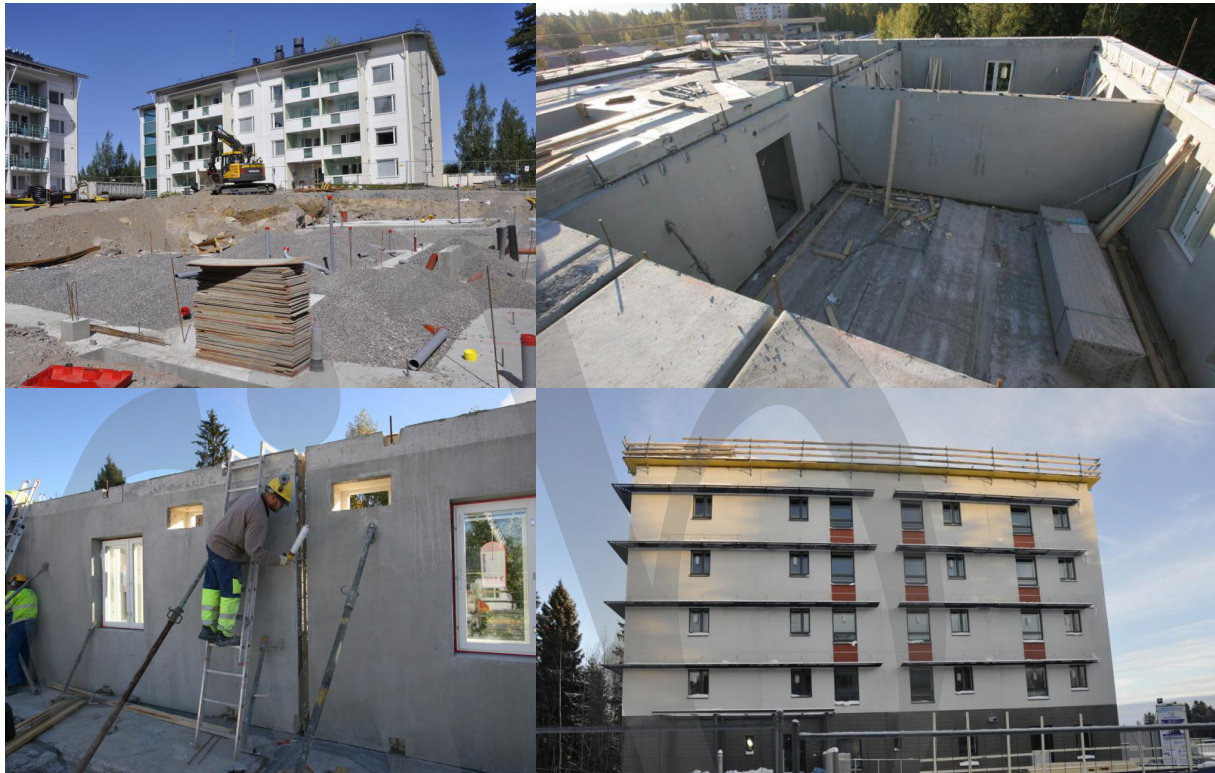
Fig. 7-2 Construction phases of the Järvenpää net zero energy building: (a) Foundations; (b) floor and intermediate walls; (c) sandwich panels and (d) Roof under construction (nollaenergia.fi)
