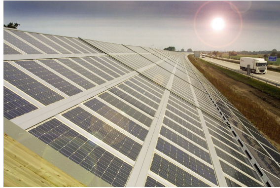
Figure 5: Solar panels alongside the highway as sound barrier.
