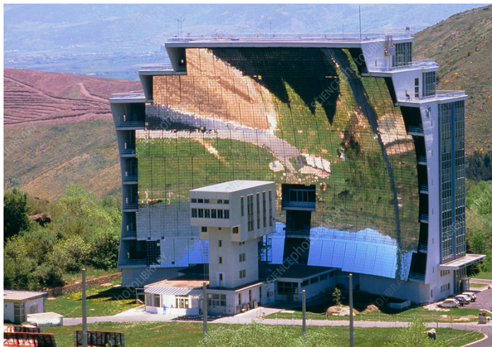
example Odeillo Solar Furnace (F)
