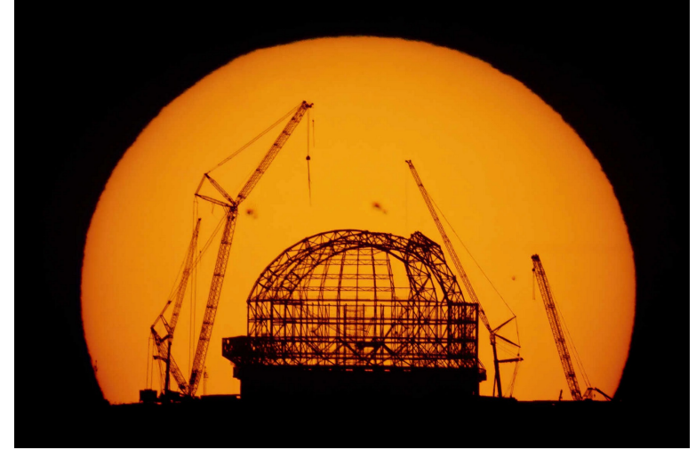
E-ELT 80 m dome construction
