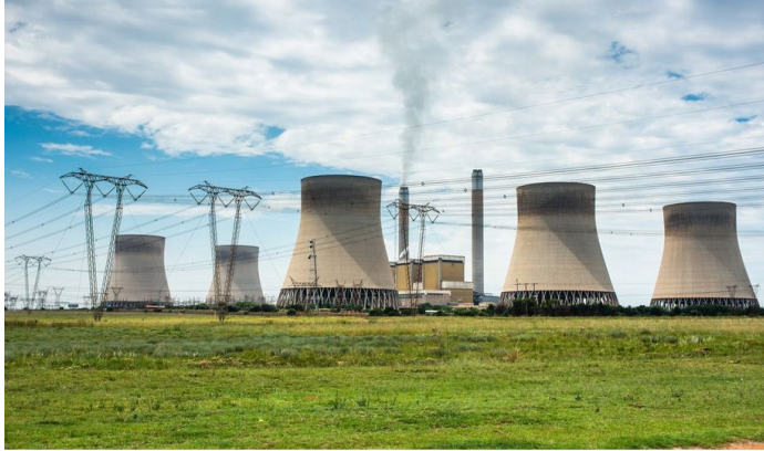
Coal-Fuelled Power Plant, South Africa
