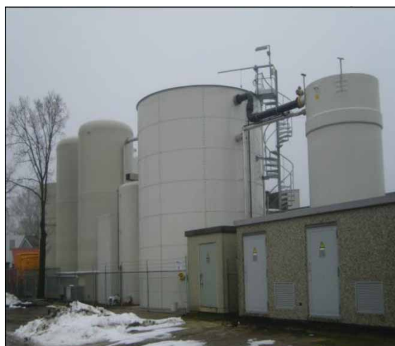
Figure 4 | Nereda ® installation – food industry.
