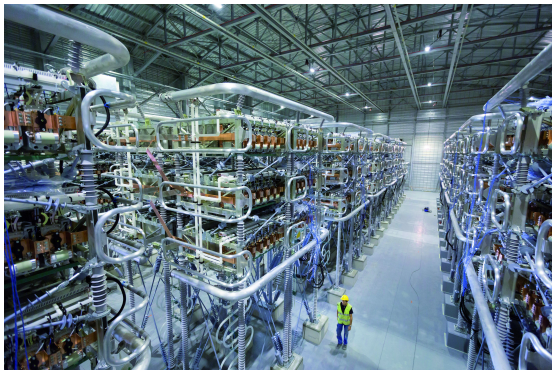
Figure 17 HVDC hall from Siemens.
