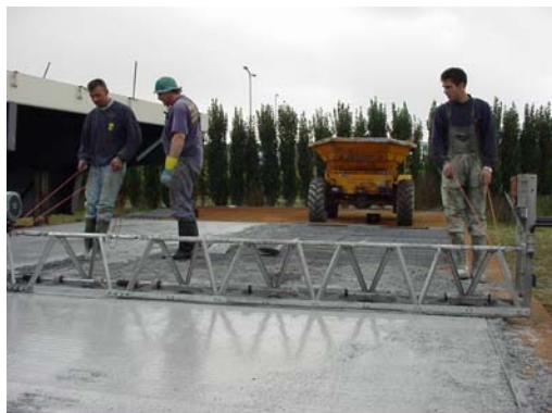
Photo 7: Placing HPC testarea.
