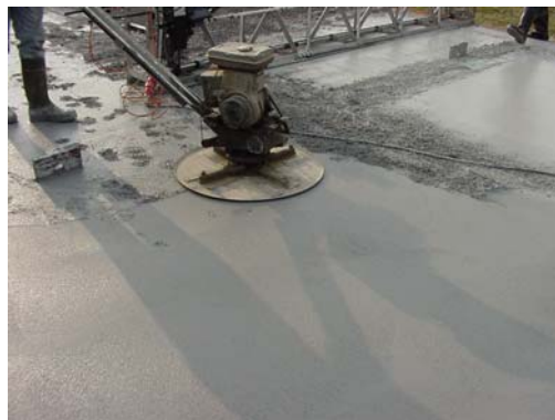
Photo 8: Finishing surface RHPC overlay.
