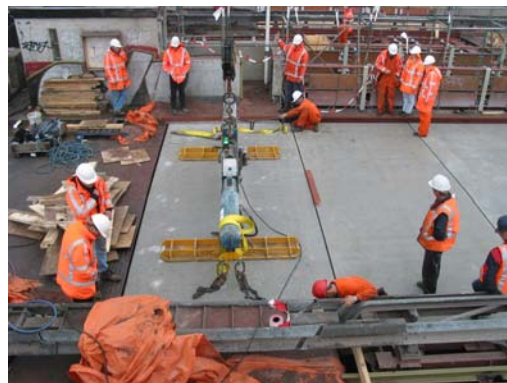
Photo 2: Placing 45 mm thick panels on a bascule bridge.
