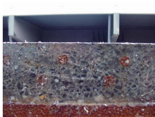
Photo 6: RHPC overlay on deck plate.
