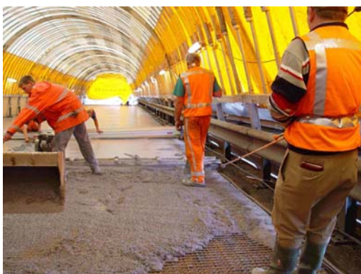
Photo 15: Casting HPC.
