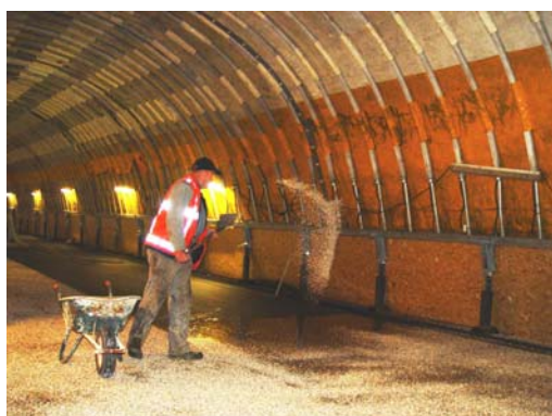
Photo 13: Placing the interface layer.
