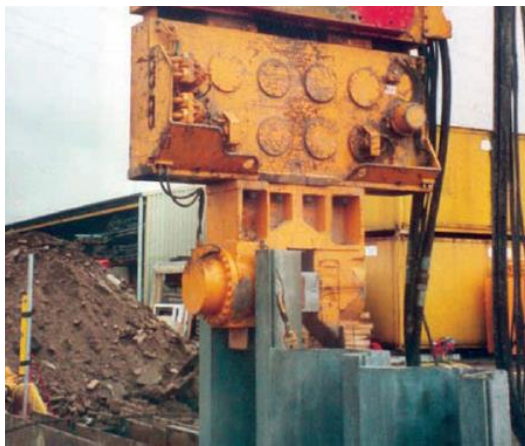
Figure 2.37: UHPFRC sheet piles being hammered
