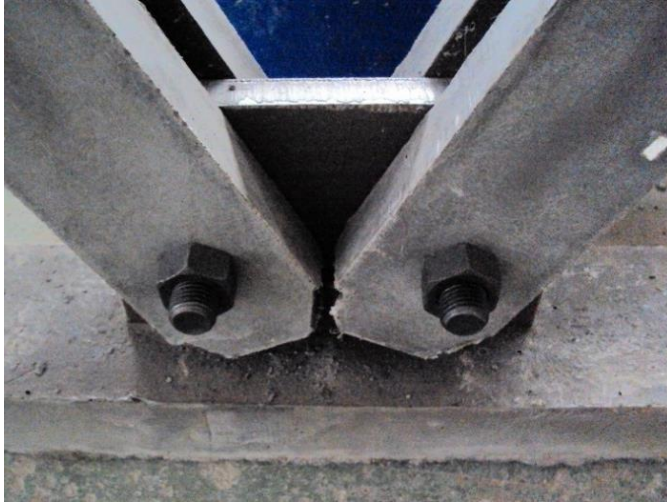
Figure 5.68: Detail of the bottom chord connection
