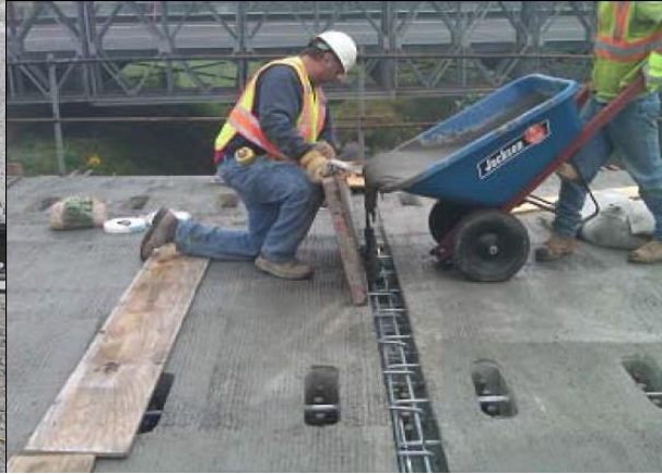
Figure 2.45: Filling the joints with UHPFRC
