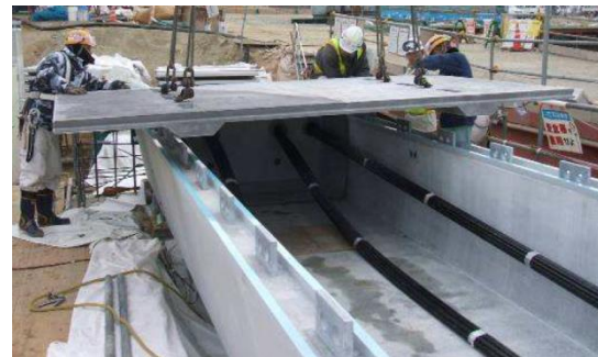
Figure 2.62: Connection between pieces
