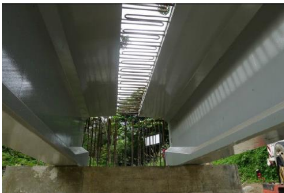
Figure 2.47: Transversal connection between the T beams
