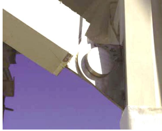
Figure 2.52: Detail of the steel bolted connection
