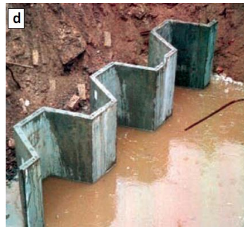
Figure 3.38: Sheet piles already placed
