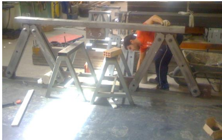
Figure 5.66: Truss during the assembly process
