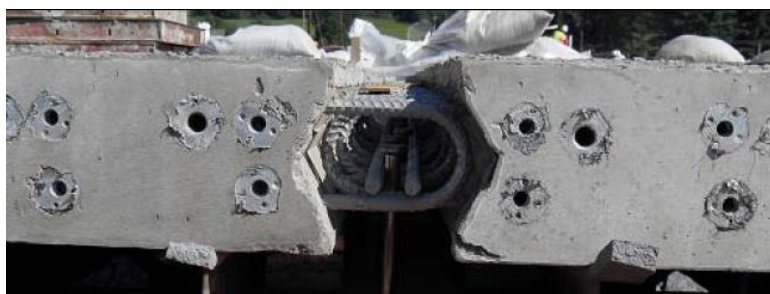
Figure 2.43: Detail of the connection between two panels
