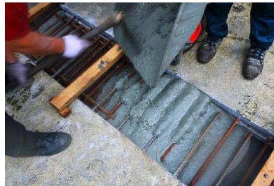
Figure 2.48: In-situ concrete being poured
