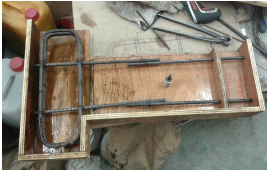
Figure 5.32: Formwork of the elements
