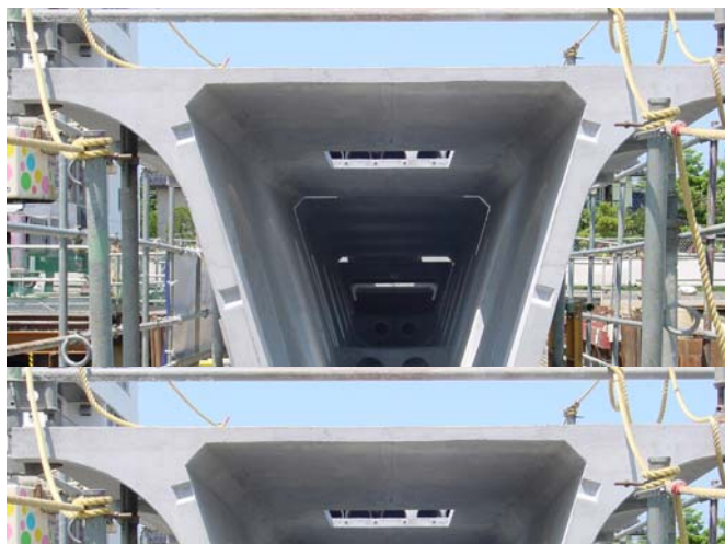
Photograph 2. Section of 1R pre-cast segment.
