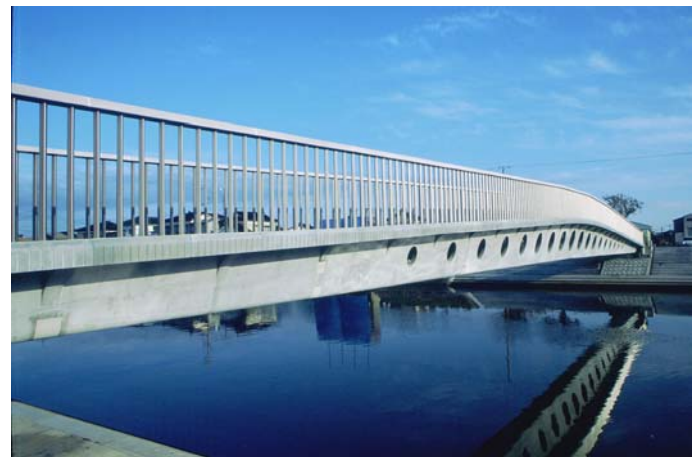
Photograph 1. Completion of Sakata-Mirai Footbridge.
