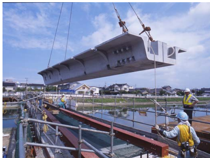
Photograph 3. Installation of 3L pre-cst segment.
