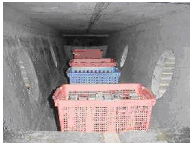
Photograph 4. Exposed specimens inside girder.
