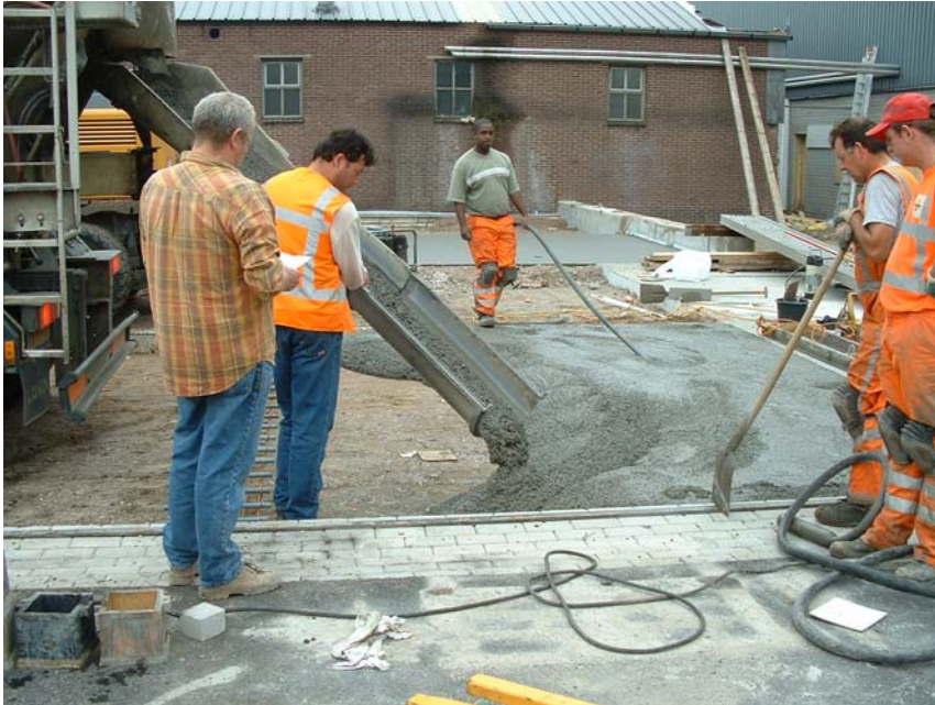
Figure 8.15 Casting and vibrating of the ecological mixture.
