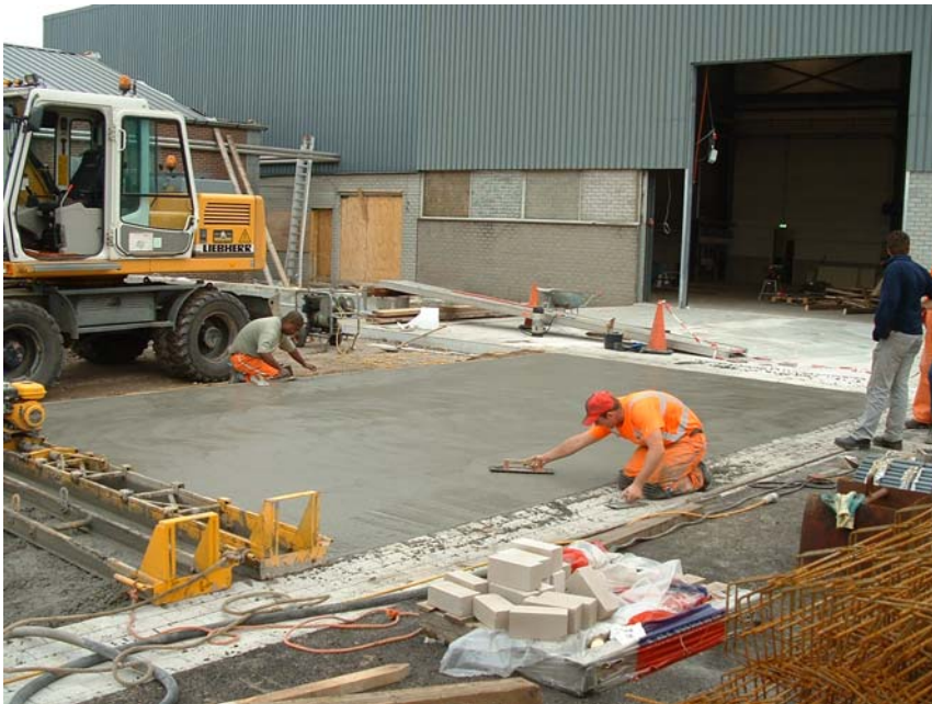
Figure 8.16 The surface of the pavements was finished between the fixed forms by two hand-operated vibratory screeds. After this, irregularities were flattened out by hand with steel floats.
