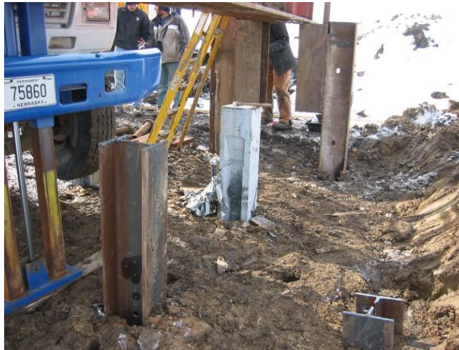
Figure 22. Photo. Experimental precast pile made of UHPC
