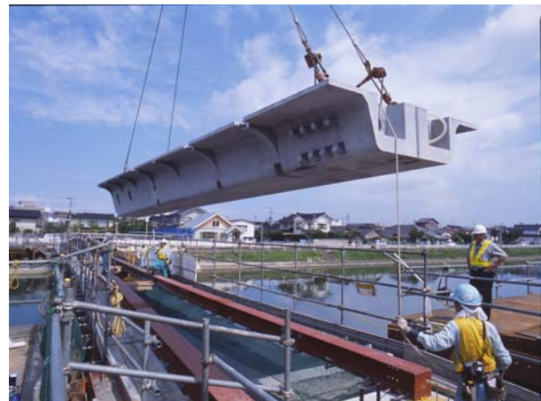
Photo 3 Installation of 3L segment
