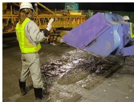
(c) Placement of HPFRCC
