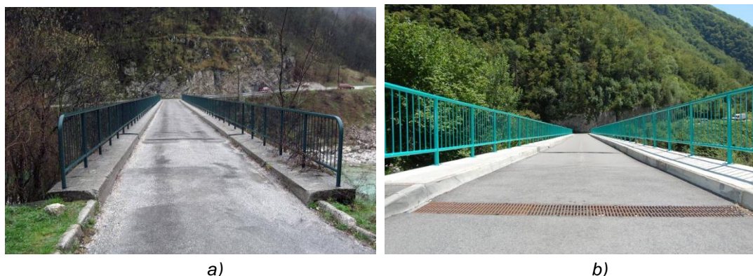
Figure 1: The Log Čezsoški bridge before a), and two years after the application of the UHPFRC layer b).
