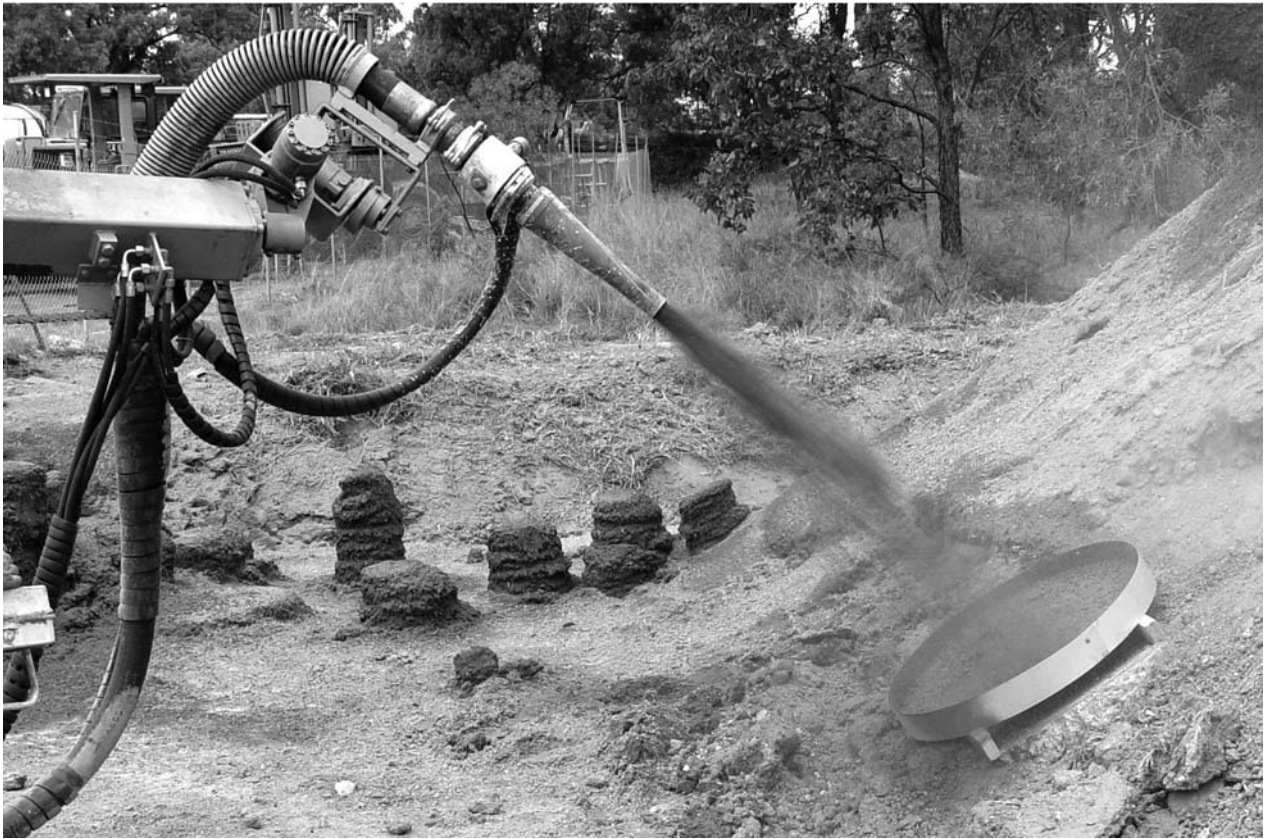
FIG. X1.6 Remotely-Controlled Spraying of Panels
