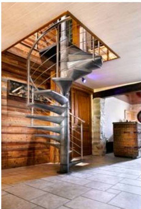
Figure 2. Stairs made of Ductal.
