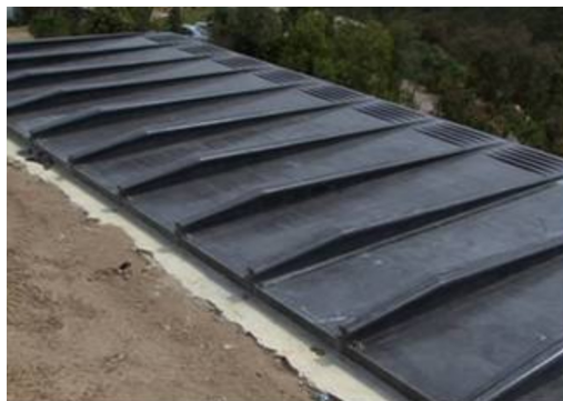
Figure 5. Ductal® roof of Navarra house.
