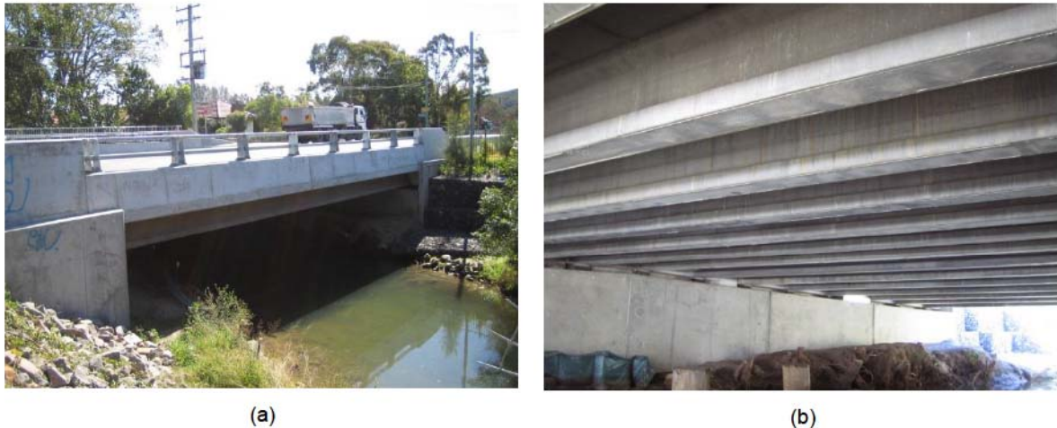
Figure 3. Shepherd's Gully Bridge, NSW, Australia constructed 2005: (a) 15 metre span 4 lane road traffic bridge (b) underside showing I-girders.
