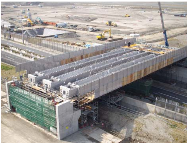
Photo 5 Erection of UFC precast blocks
