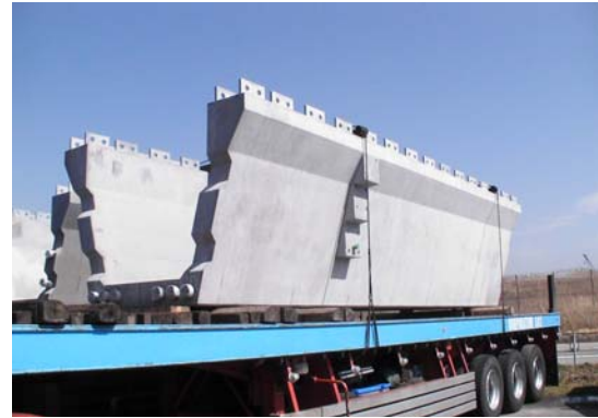
Photo 1 UFC precast block
