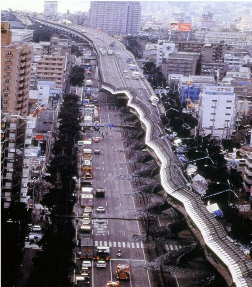
Overtaken Hanshin Expressway, 1995 Kobe Earthquake, Japan (images courtesy of AIJ)
