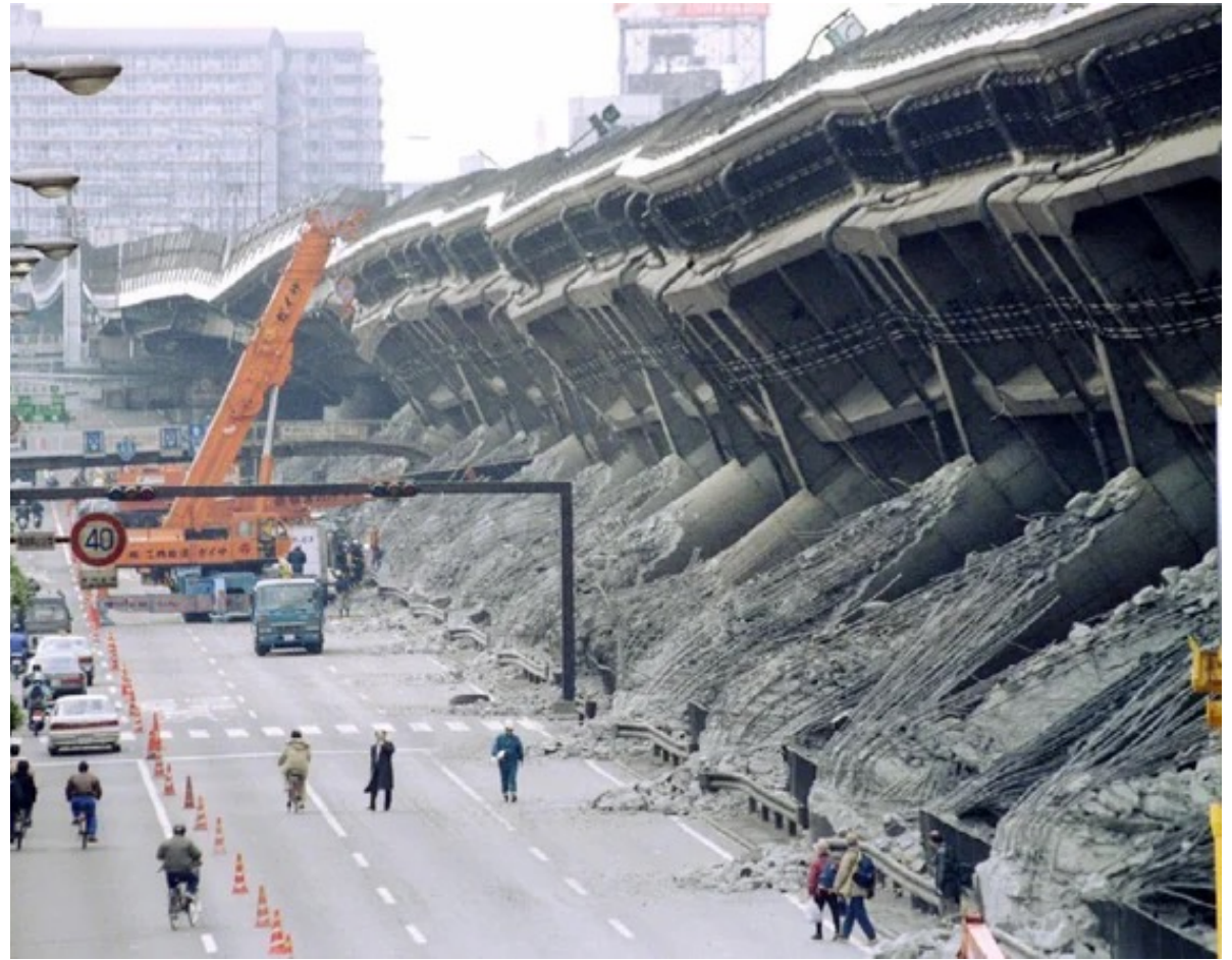
Overtaken Hanshin Expressway, 1995 Kobe Earthquake, Japan (images courtesy of AIJ)
