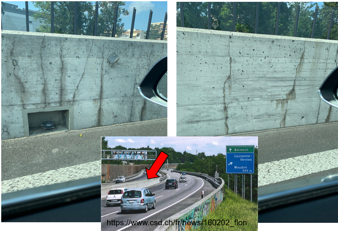
Arch bridge over le Flon, A9, lakeside exit Lausanne - Vennes
