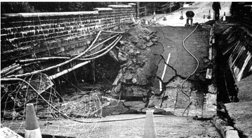
1.6 Collapse of the Ynys-y-Gwas bridge led to a ban on grouted tendons. 17
