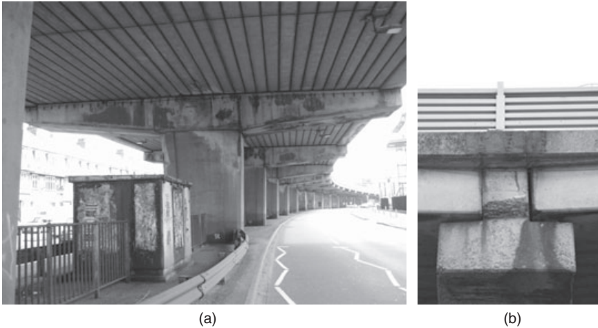
1.5 M4 viaduct in west London: (a) corrosion problems are apparent, and (b) the leaking joint above the crosshead beam. 11
