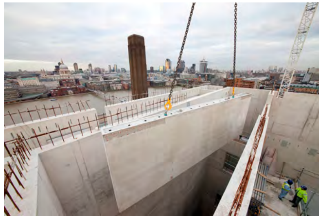
Fig. 7-8: Installation of a solid wall inside an insitu core.
