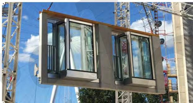
Fig. 9-8: Punched panel with two glazed "winter gardens" (courtesy of Explore Manufacturing UK).
