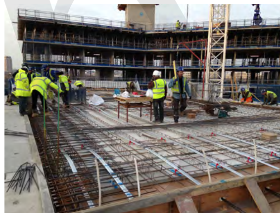
Fig. 5-10: Post tensioning sheaths fixed above filigree slab.
