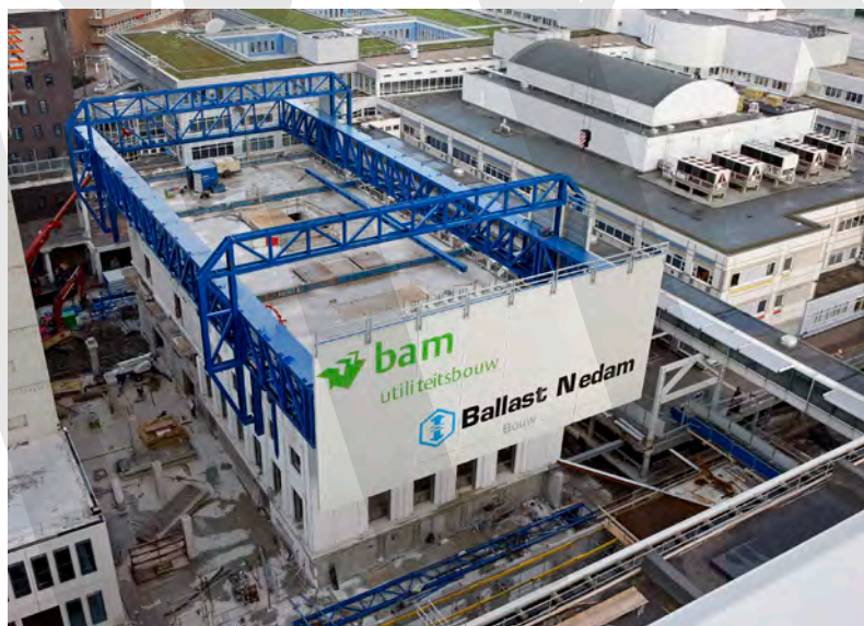
Fig. 11-9: Hoisting Shed Assembly, courtesy of BAM.
