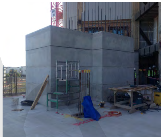
Fig. 3-8: Twin shaft produced as complete plan section with horizontal joints only.
