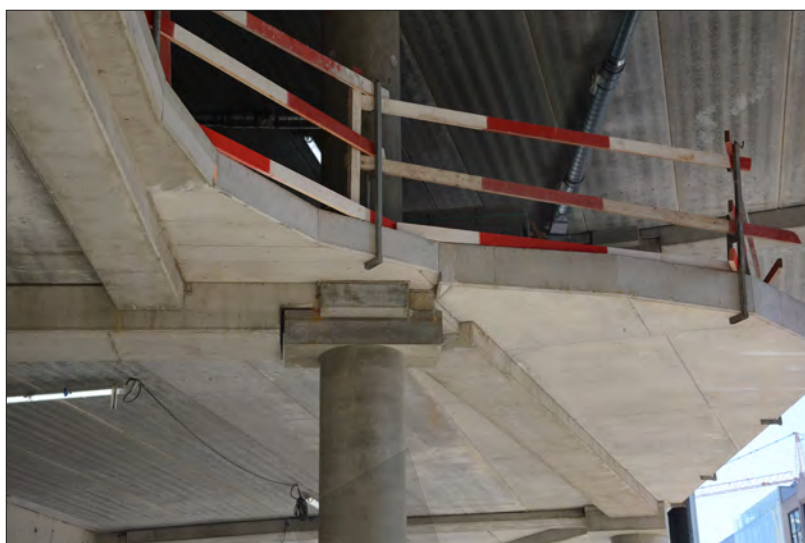
Fig. 6-31: Example of Type A connection at irregular slab edge.
