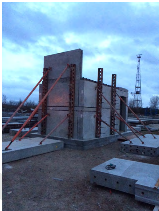
Fig. 2-11: Prototype storey height precast walled core and stairs for Battersea PowerStation Development, London.
