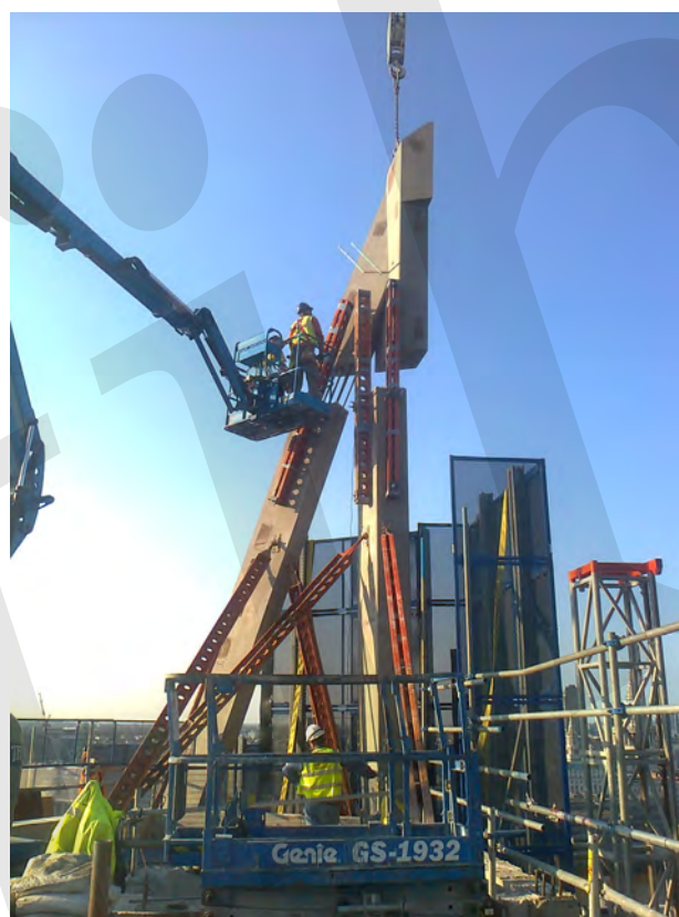
Fig. 2-8: Corner column completed at roof level, Blackfriars, London.
