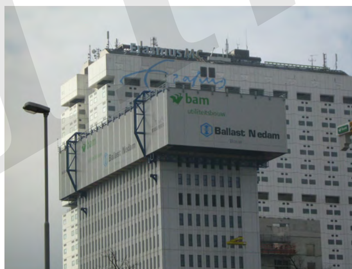
Fig. 11-8: Example of Hoisting Shed, courtesy of BAM.
