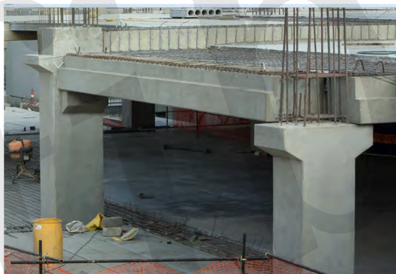
Fig. 6-32: Example of Type B connection. Insitu stitching to be provided between columns and supported beams at corner connection (Embassy 7B project, Bangalore, India, courtesy of KEF Infrastructure Pvt Ltd).
