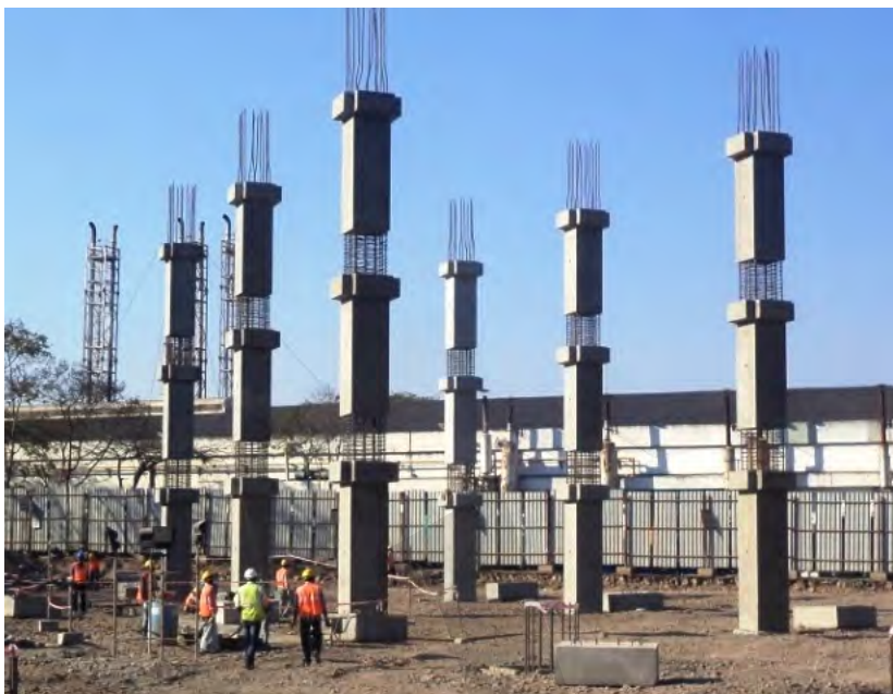
Fig. 4-3: Multi storey columns with gaps to allow for connection at floor levels (courtesy of Precast India Infrastructures Pvt Ltd, from fib Bulletin 78 15 ).
