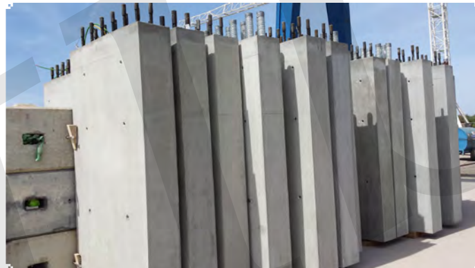
Fig. 7-15: Stored precast wall panels with mixture of top connectors.
