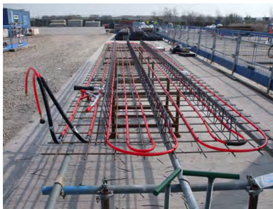
Fig. 5-7: Coolant pipes tied to bottom reinforcing mesh.
