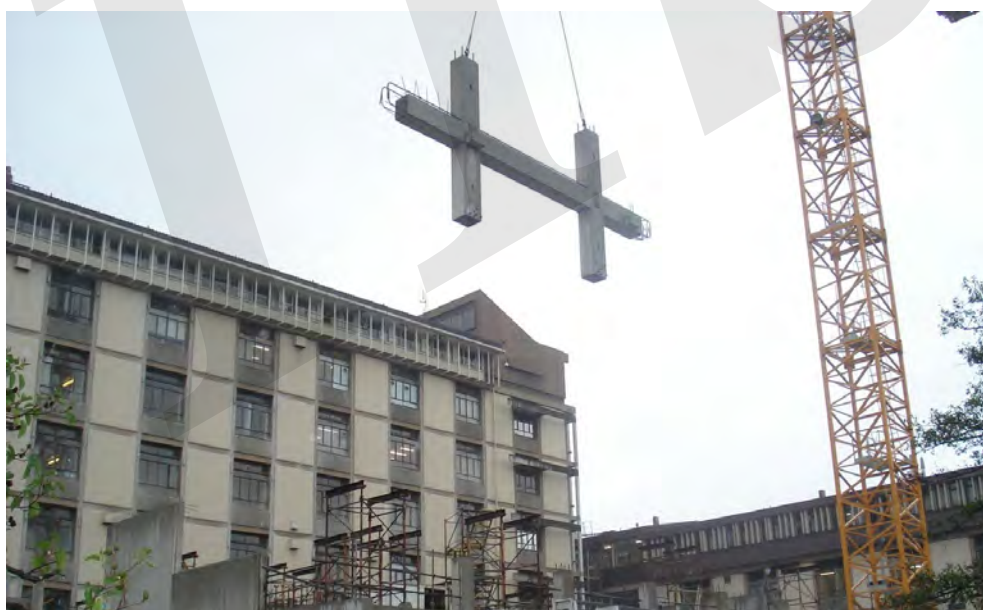
Fig. 4-4: Sub-frame with connections at mid lengths of columns and beams (Biological Science Building under construction at University of Canterbury Campus, New Zealand, photo courtesy of Stefano Pampanin).
