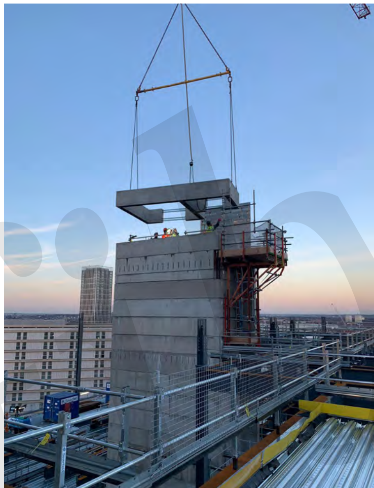
Fig. 11-2: Lifting Arrangement for Double Shaft Segments.
