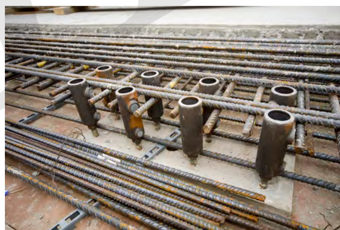
Fig. 6-29: Couplers fixed to top of precast column at construction site.
