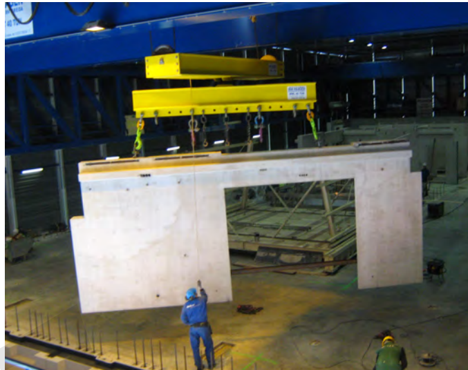
Fig. 12-11c: Horizontal distribution of precast panel inside climbing shed.
