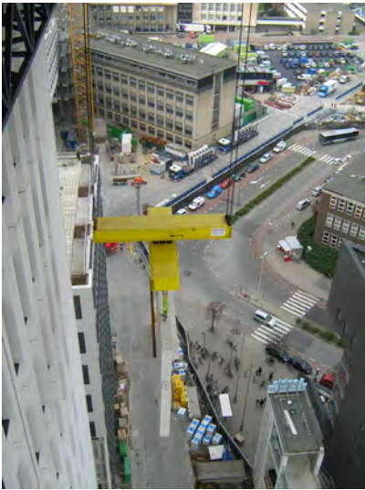
Fig. 12-11b: Vertical lift of precast panel from delivery vehicle.
