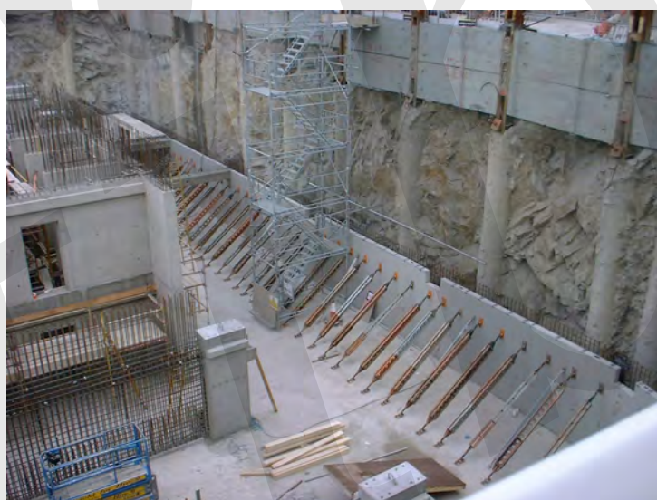
Fig. 2-7: Precast basement perimeter wall and high strength columns, Dublin, Ireland.
