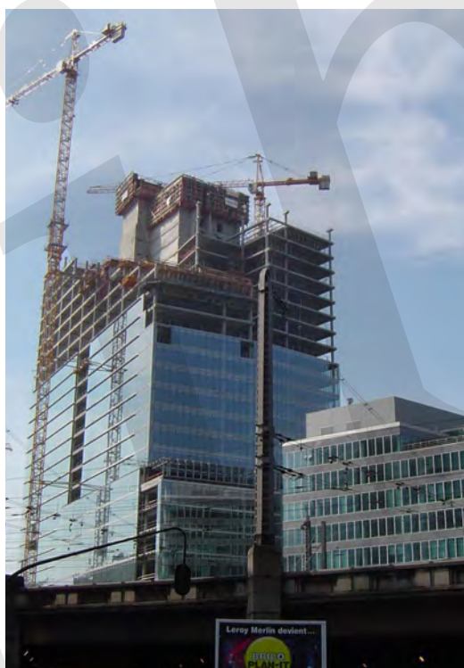
Fig. 3-4: North Galaxy, Brussels. Columns and beams as shown in Figure 3.3 with insitu stability core.
