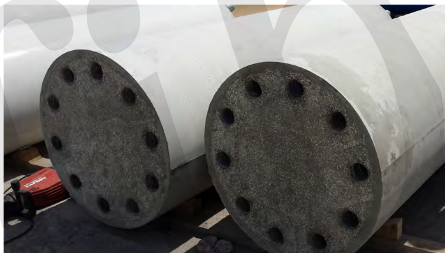
Fig. 6-2: 900 mm diameter single storey circular columns with cast in tubes for connections at floor levels.
