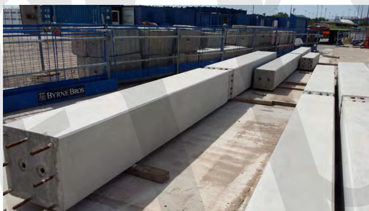
Fig. 6-13: Horizontally cast double storey square columns with intermediate coupler connection for floor slab.
