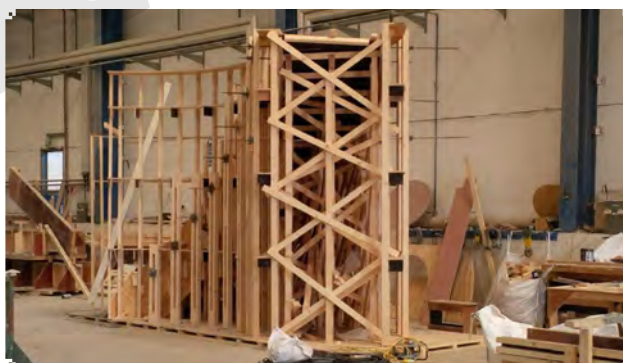
Fig. 8-24: Timber Ramp mould used for helical flight.
