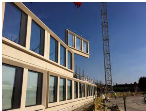
Fig. 9-7: Punched panel with three pre fixed windows (courtesy of Explore Manufacturing UK).
