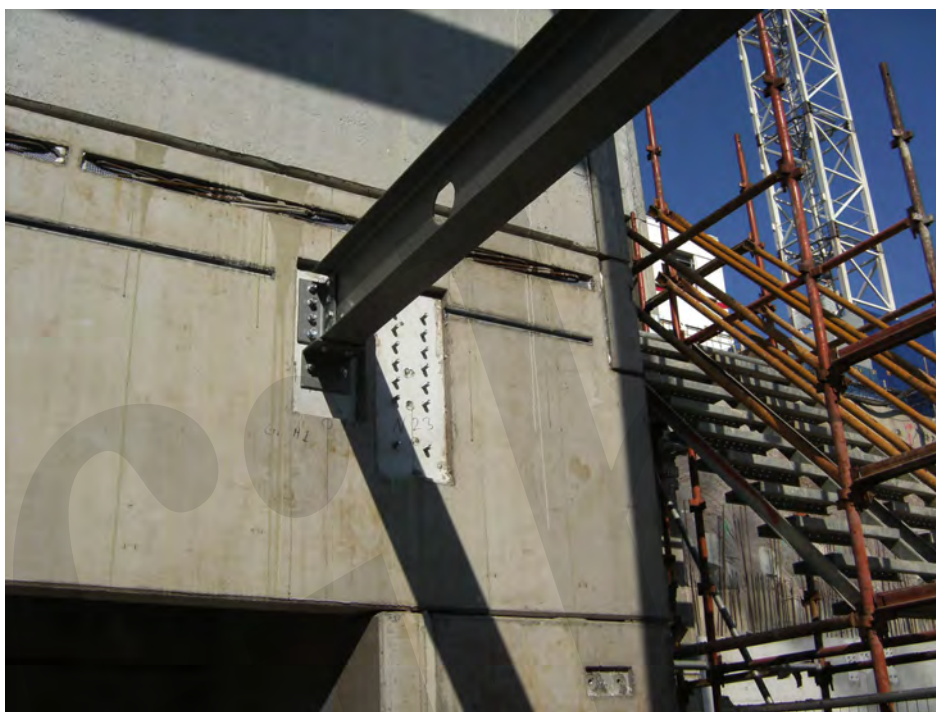
Fig. 3-15: Example of connection of steelwork to precast concrete core.
