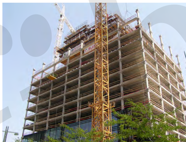
Fig. 6-20: Double storey circular columns installed in the building frame.
