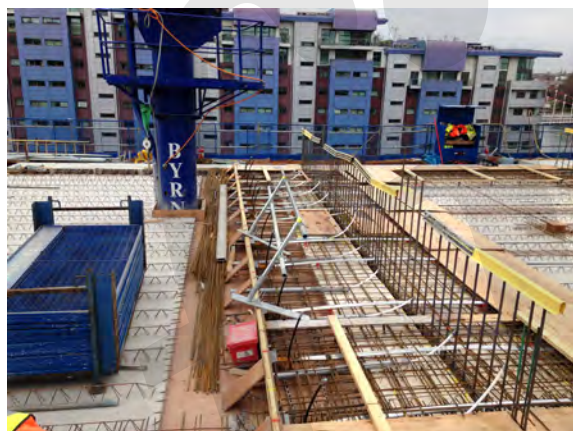
Fig. 5-9: End anchorage in post tensioned filigree slab system.
