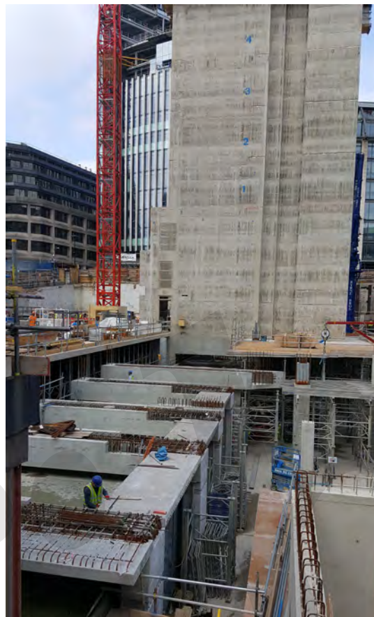
Fig. 3-17: Precast concrete U beams bridging existing structure, note precast panel in background supporting slipformed core.
