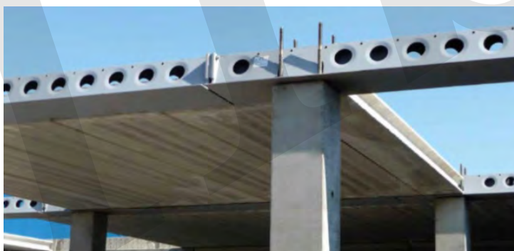
Fig. 5-18: Proprietary steel DELTABEAM® and hollowcore slabs providing flat soffit through “slim-floor” system, courtesy of ©Peikko Group Corporation.
