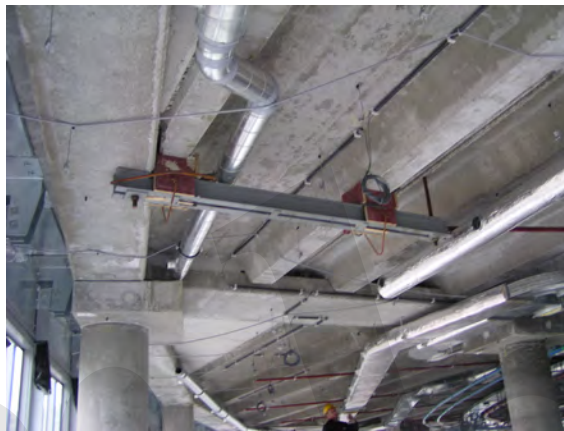
Fig. 5-13: An example of fixing services beneath a double tee ribbed floor.
