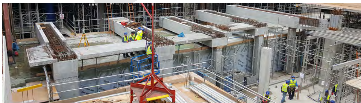
Fig. 2-6: Precast U beams and slabs at a transfer level.
