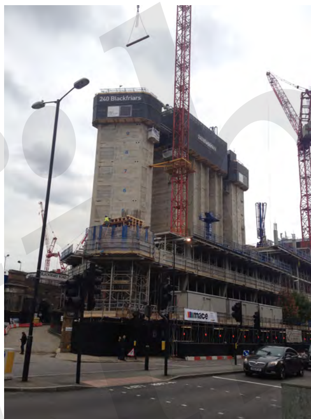
Fig. 3-1: Slipformed concrete cores at Blackfriars, London.
