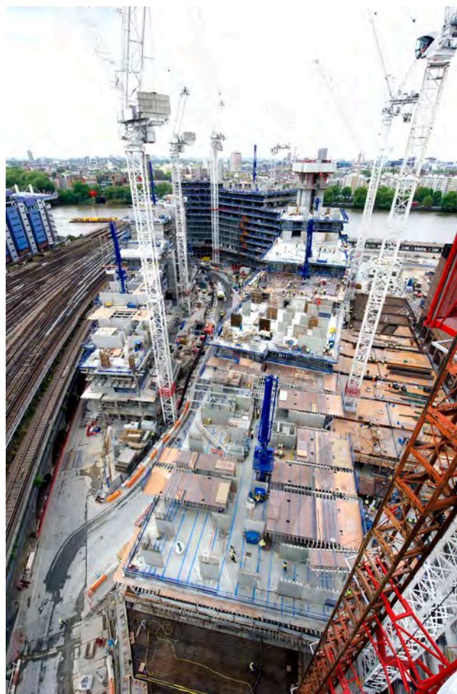
Fig. 3-5: Battersea Power Station Residential Development, London (Example of precast concrete columns and walls with post tensioned insitu slab, courtesy of Byrne Brothers(Formwork) Ltd.
