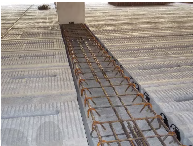
Fig. 3-11: Prestressed precast beam intended for composite action and moment continuity.
