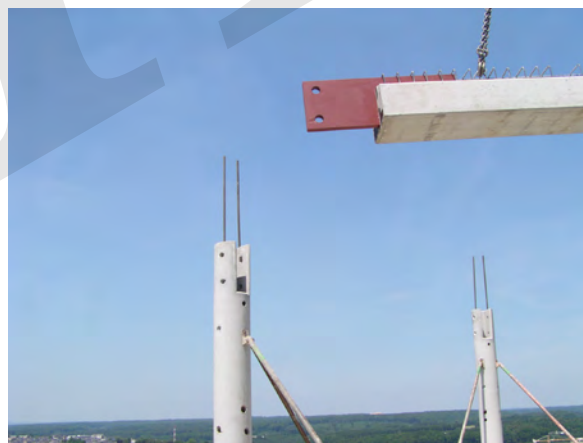
Fig. 6-34: Beam with steel connector being installed onto precast columns.
