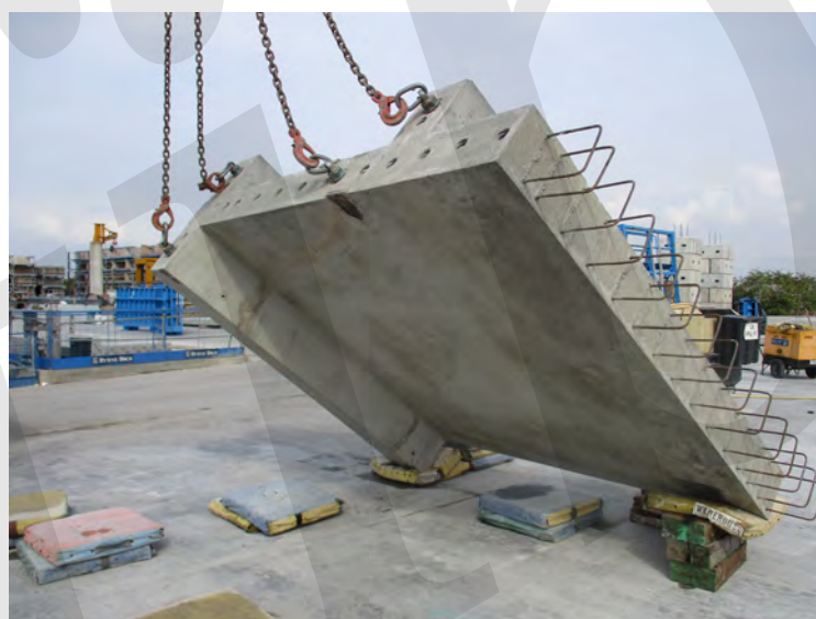
Fig. 7-3: Precast element forming part of composite wall for integrated lift shaft and stair core. Corners with adjoining walls are provided in the precast element with projecting reinforcement for connection to other structure.
