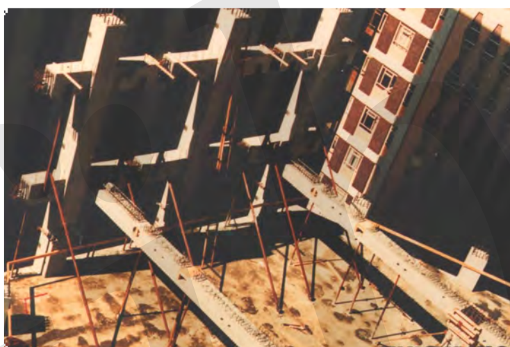
Fig. 10-6: Multi storey columns and beams in emulative system, Unisys House, Wellington, New Zealand, courtesy of A.O'Leary, from fib Bulletin 27
