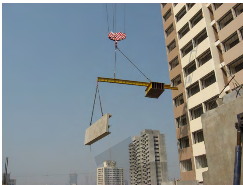
Fig. 11-3: Counterbalanced Lifting System.
