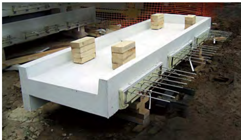
Fig. 2-14: Cantilever balconies with structural thermal break.
