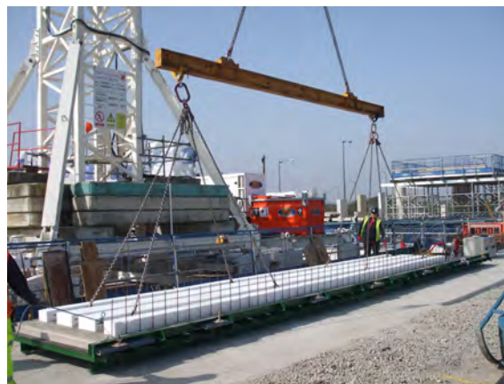
Fig. 5-8: Long span slab with solid void formers, lifted at several points.
