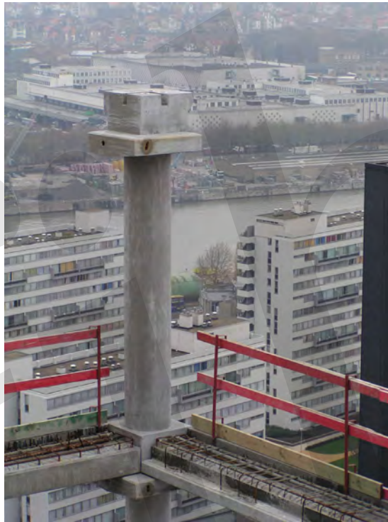
Fig. 6-30: Example of Type A connection at corner column.
