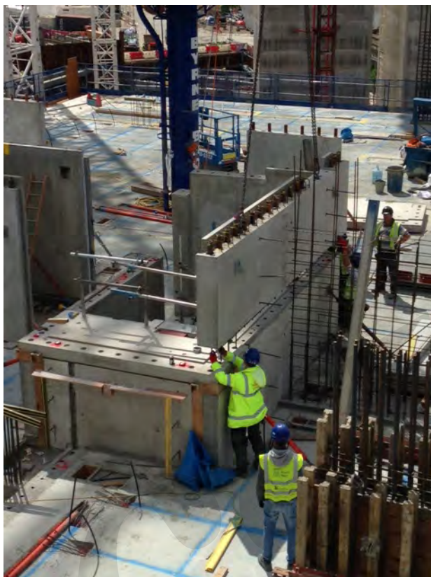
Fig. 3-7: Example of precast concrete staircore using flat panels.
