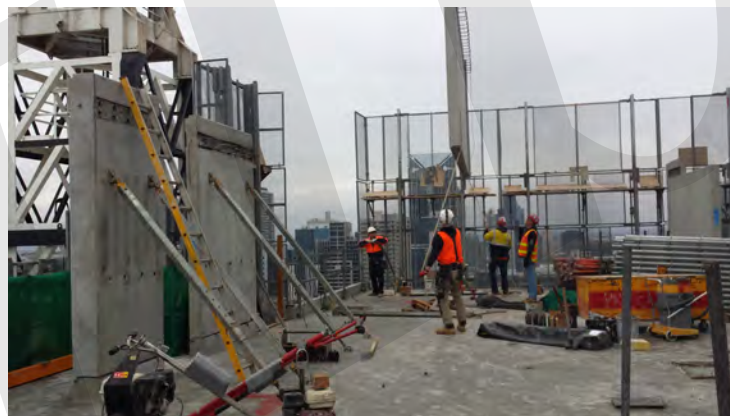
Fig. 11-6: Example of Temporary Propping and Installation of Wall Panels.
