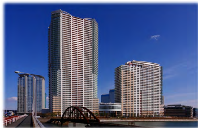
Fig. 4-5: Building with precast moment resisting frames in Tokyo (SQRIM system, refer also to case study 12.5).
