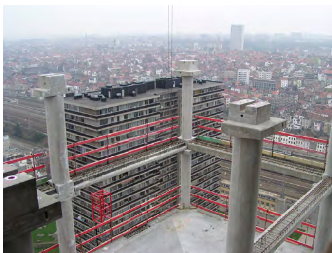
Fig. 3-3: Precast concrete double storey columns and prestressed beams, Brussels (Note insitu concrete topping to complete floor diaphragm).
