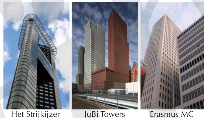
Fig. 4-11: Ex. of buildings in the Netherlands constructed using precast concrete wall systems for lateral stability.
