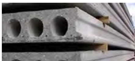
Fig. 5-16: Slab longitudinal edge profile and end transverse section.
