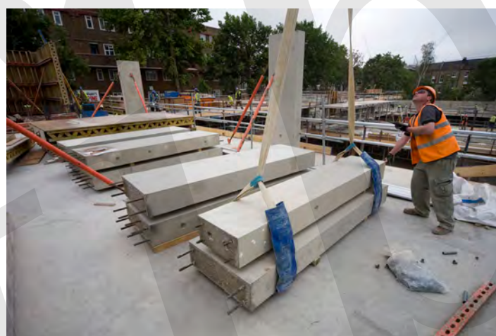
Fig. 6-28: Short projecting bars at ends of precast columns with grouted couplers.
