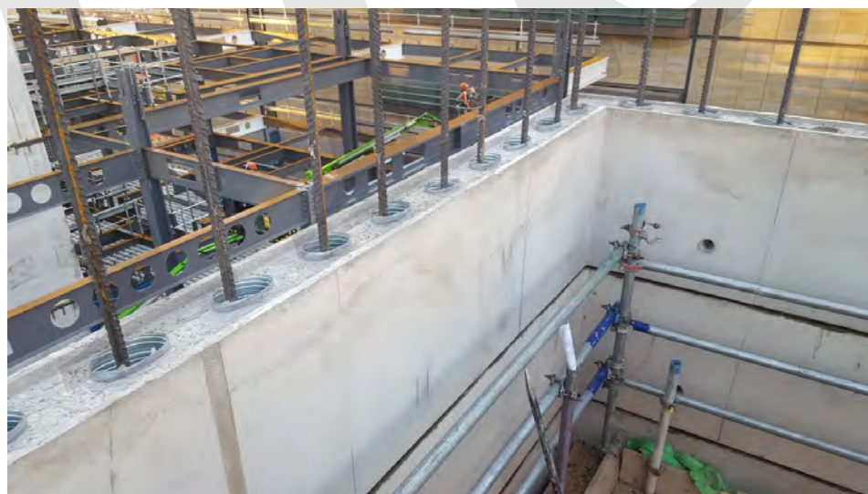
Fig. 11-4: Connecting Vertical Bars at Horizontal Wall Joint.
