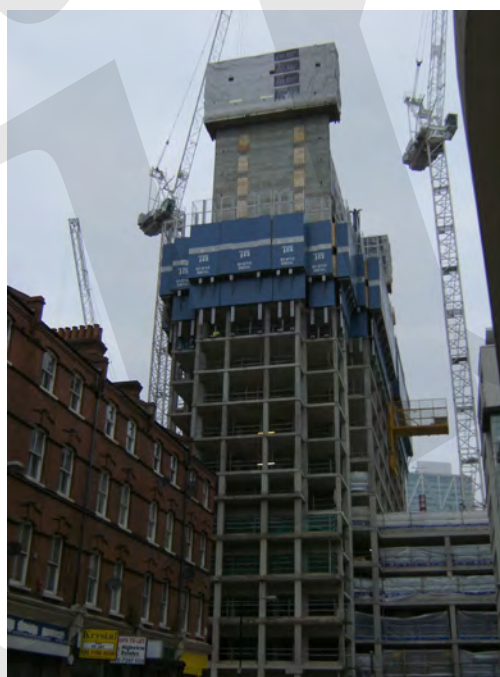
Fig. 2-1a: Nido Spitalfields, London, using precast concrete blade columns.
