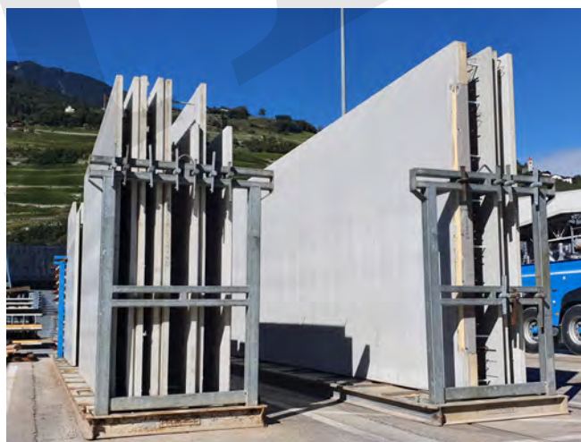
Fig. 7-21: Vertically stored wall panels on steel framed platforms.
