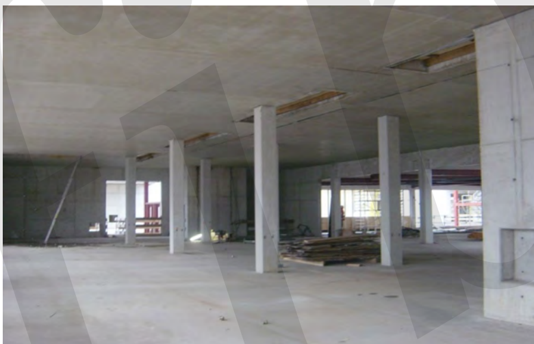
Fig. 3-9: Flat slab solution using Airdeck precast slabs composite with an insitu topping, courtesy of Airdeck Building Concepts nv.
