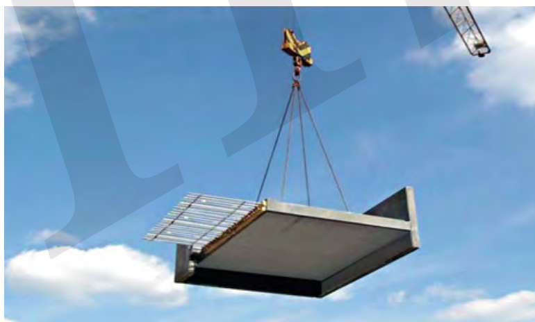
Fig. 2-13: Precast balcony with large edge upstand.
