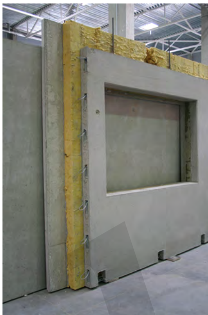
Fig. 2-5: External sandwich panel after production.
