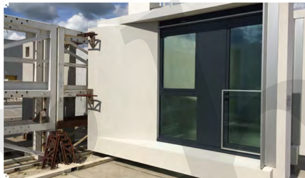
Fig. 9-2: External precast panel with windows (courtesy of Explore Manufacturing UK).
