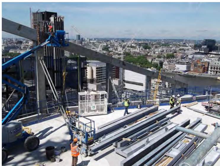
Fig. 2-9: Edge roof beams rising to meet corner column in Fig. 2-8.
