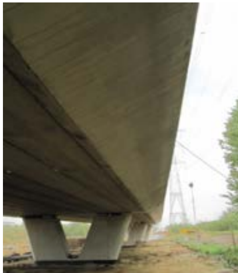
Fig. 5-16 Photo of the bridge that shows the overhang formed by the edge U girder.
