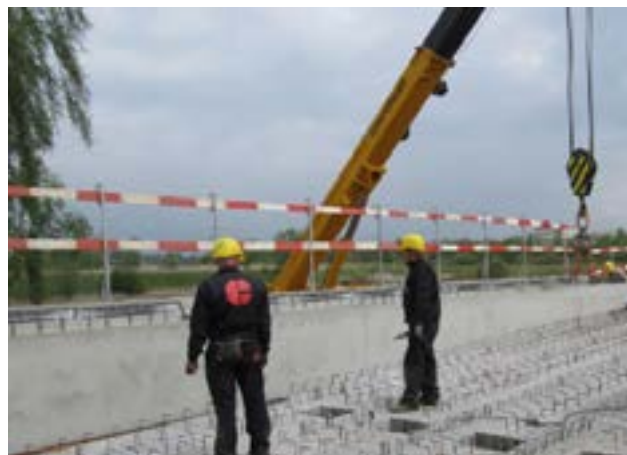
Fig. 5-27 Top flanges of girders just before installation of slab reinforcement. Holes in flanges provide access to place intermediate diaphragm connection concrete.
