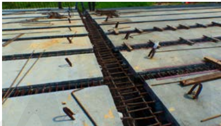
c) Example of typical diaphragm pier connection
