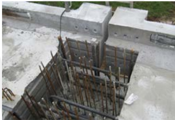
Fig. 5-22 Typical reinforcement extending vertically from the precast concrete pier beam.
