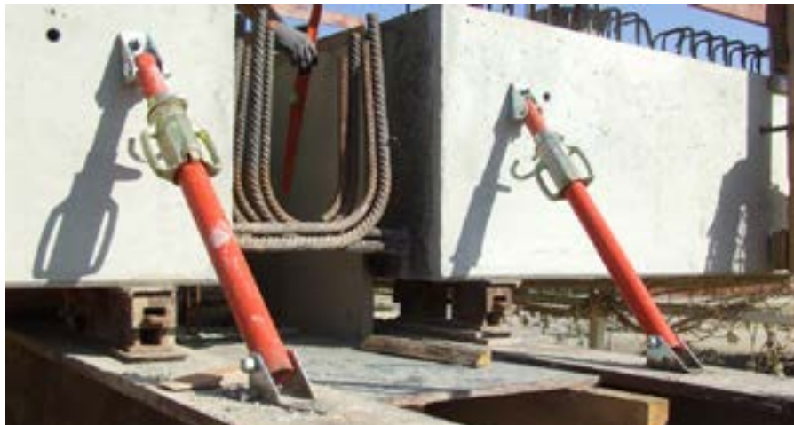
Fig. 5-107 Example of bottom positive moment continuity reinforcement in a bridge girder.
