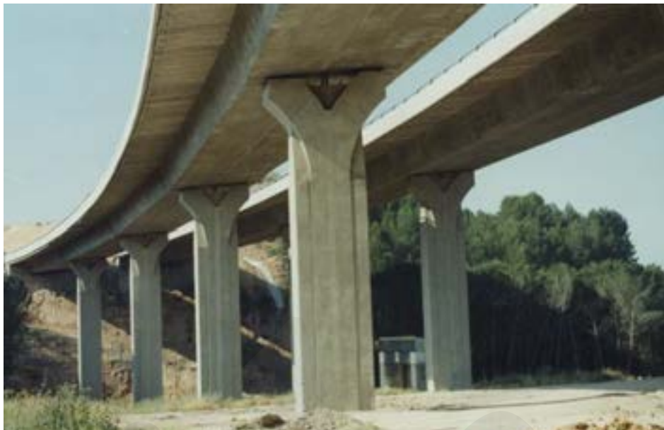
Fig. 4-2 Precast concrete superstructure with curved concrete girders [4-7] Source: fib Bulletin 29, Precast concrete bridges (Lausanne, Switzerland: International Federation for Structural Concrete, 2004).
