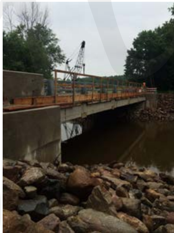
Fig. 5-258 Subsequent beams are installed.
