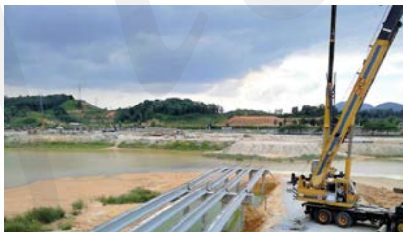
c) Example of Installation of girders on abutment
