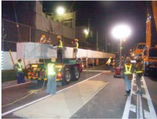
Fig. 5-131 Transporting the precast concrete girder by truck.
