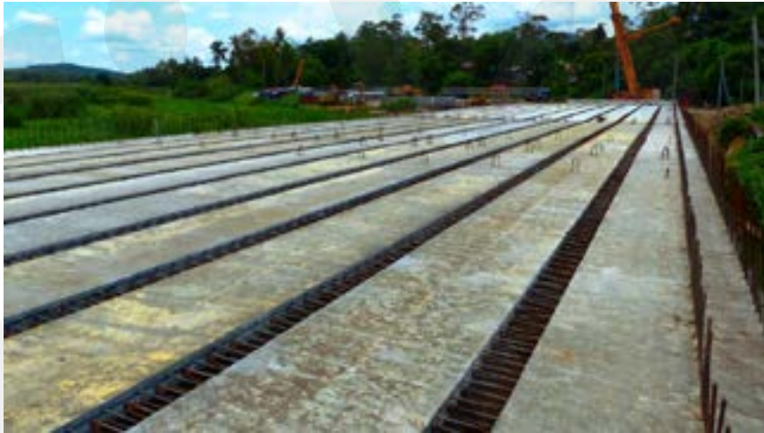
Fig. 5-190 Final positioning of the last edge girder.
