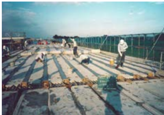
Fig. 5-133 Concrete is being placed between precast concrete girders and will be followed by casting concrete in the diaphragms.
