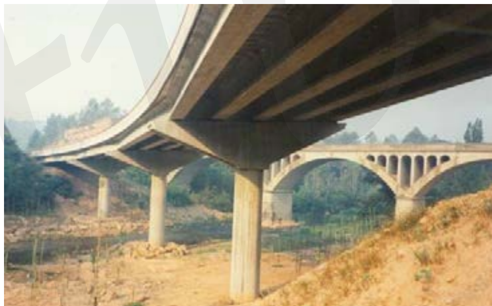
Fig. 4-1 Precast concrete superstructure with chord length concrete girders [4-7] Source: fib Bulletin 29, Precast concrete bridges (Lausanne, Switzerland: International Federation for Structural Concrete, 2004).
