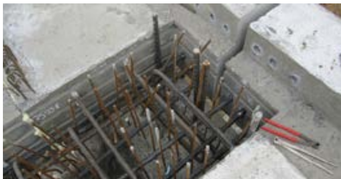
Fig. 5-23 Another view of the continuity reinforcement extending from the pier cap and dapped ends of the U girders.
