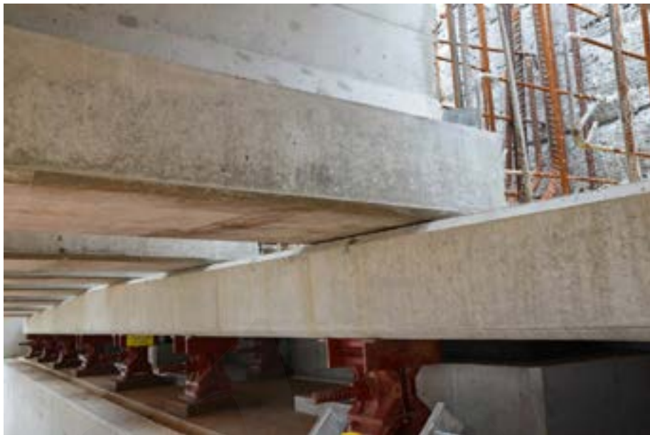
Fig. 5-109 Transverse precast concrete soffit beam and mechanical supports.
