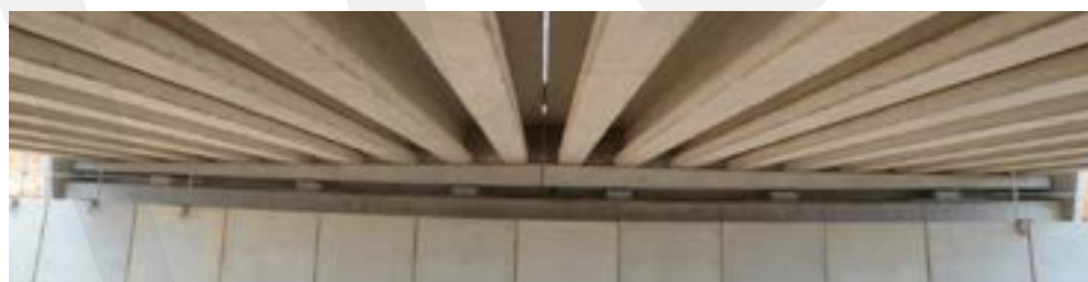
Fig. 5-99 Example of a precast concrete soffit beam with transverse slope.
