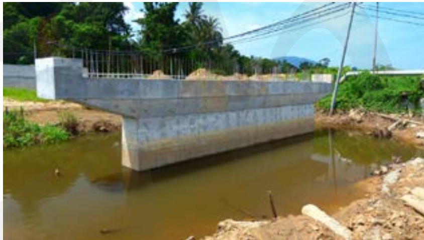
Fig. 5-185 An example of typical pier and pier cap ready for installation of girders.
