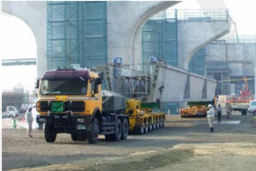
Fig. 5-155 Transporting a precast concrete girder fabricated at the jobsite.
