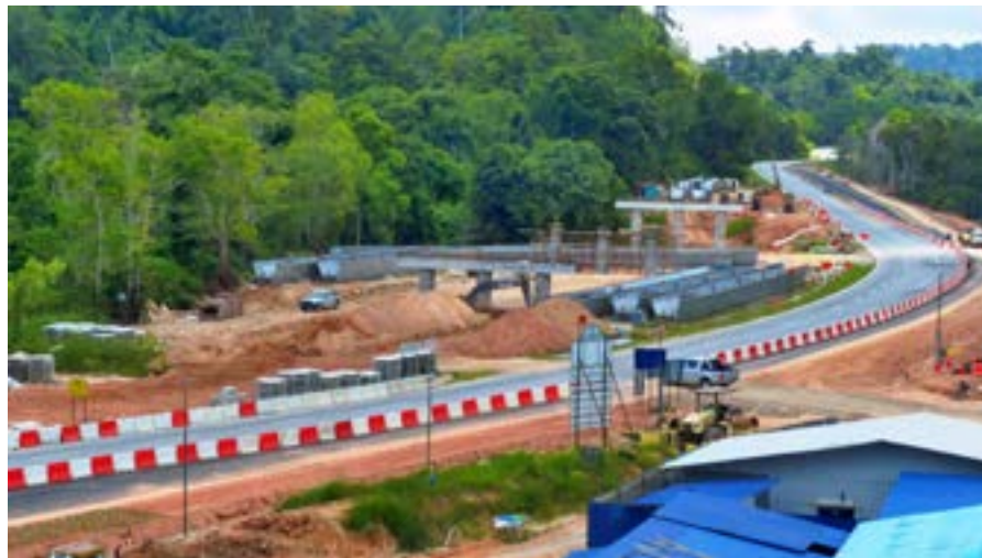
Fig. 5-208 Another view of piers with girders awaiting erection. Girders have begun to be set in the background.
