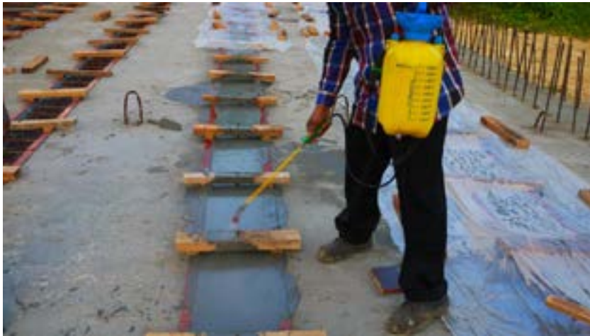
Fig. 5-195 Application of curing compound.
