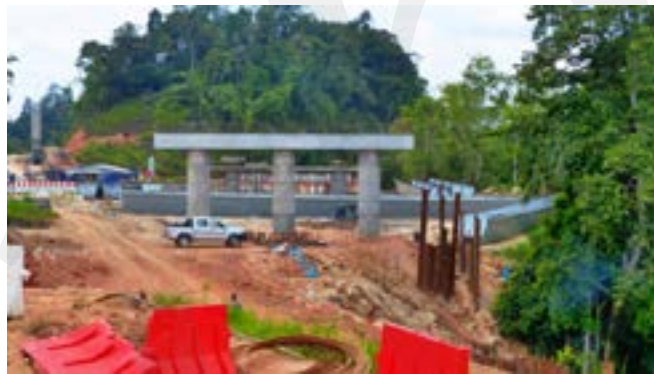
Fig. 5-207 Forms for the construction of the pier beam have been removed. Girders are staged nearby ready to be put in place.
