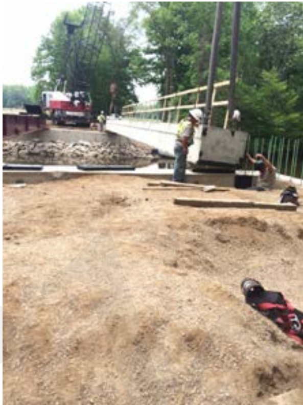
Fig. 5-257 Erection of the first edge beam.
