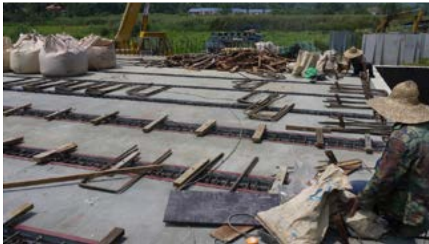
Fig. 5-192 Edges of the flanges are shown here having been protected, bottom forms are suspended from the wooden strong backs, and reinforcement is at the ready to extend from the joints at the ends.
