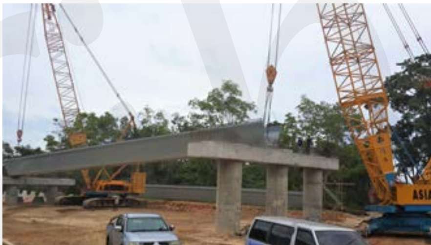
Fig. 5-209 These U girders require two cranes for erection.
