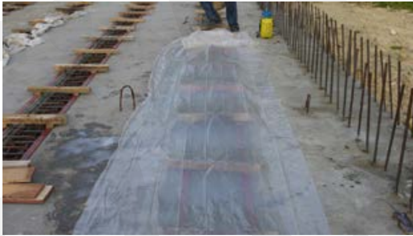
Fig. 5-196 Applying curing cover.
