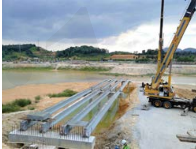
Fig. 5-166 Example of precast girder installation
