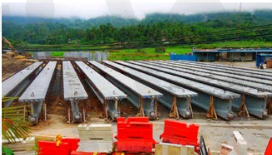
Fig. 5-188 Girders in temporary storage. Shores under flanges ensure stability.
