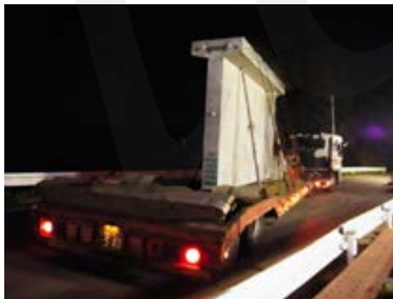
Fig. 5-144 Transportation of a precast concrete girder segment by truck.
