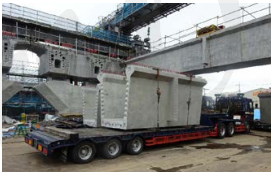
Fig. 5-153 Transporting the U girder segments.
