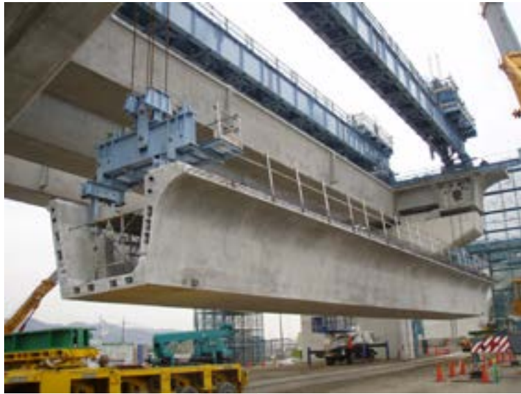
Fig. 5-154 Erection of the U girder. The post-tensioning ducts and anchorages are seen at the end.
