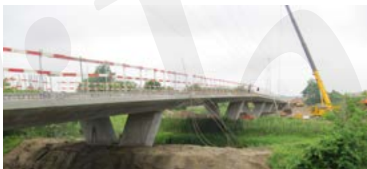
Fig. 5-28 Elevation view of the bridge before casting deck slab.
