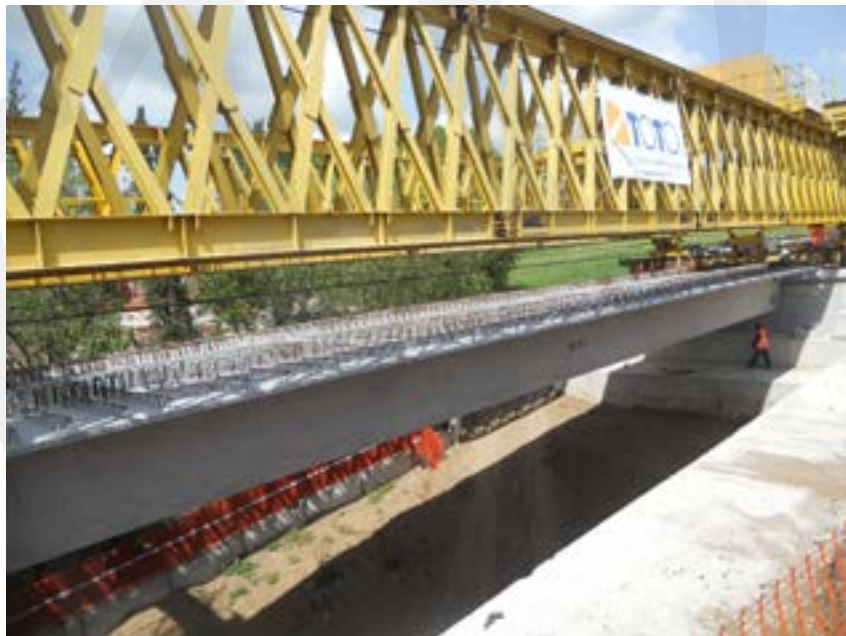
Fig. 5-122 Launching the U girder under a trussed steel launching beam.
