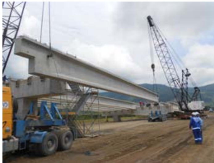
Fig. 5-73 Transporting and installing girders.
