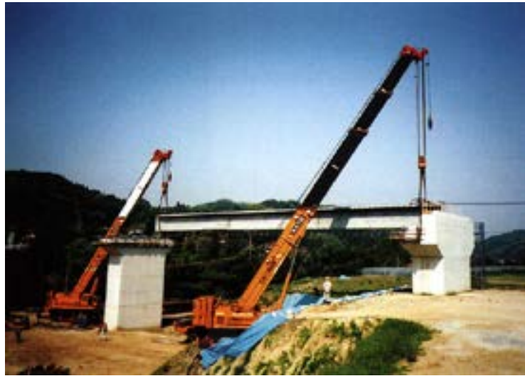
Fig. 5-142 Erection using two-point picks with two cranes.
