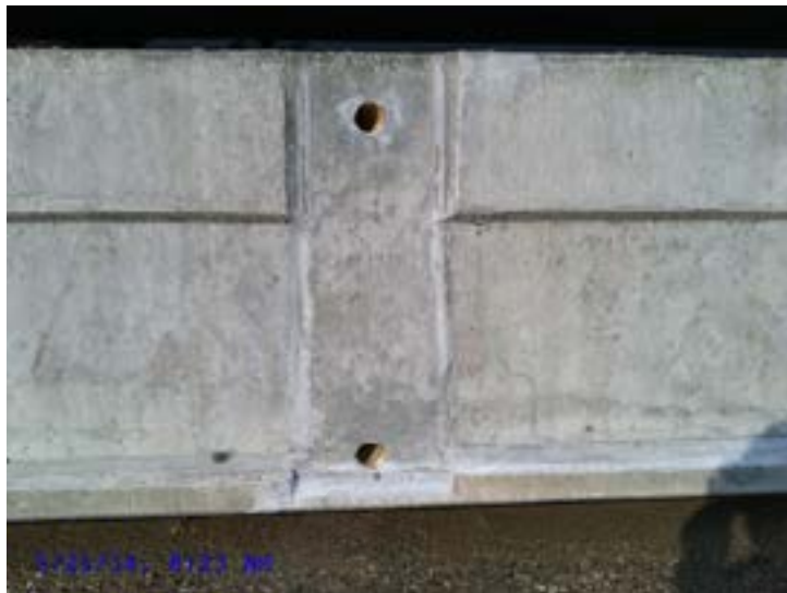
Fig. 5-256 Vertical and horizontal shear keys at the post-tensioning location.
