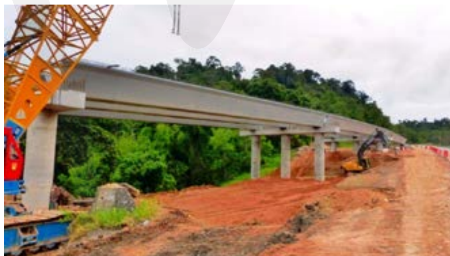
Fig. 5-210 This bridge, like the example bridge, has three girders in the cross section and vertical curvature.
