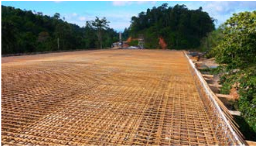
Fig. 5-211 Edge forms for the deck and curb have been built and reinforcement placed awaiting casting of the deck concrete.
