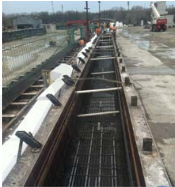
Fig. 5-254 Partial reinforcement setup in a beam form before concrete placement. Top and bottom PVC post-tensioning ducts are visible.
