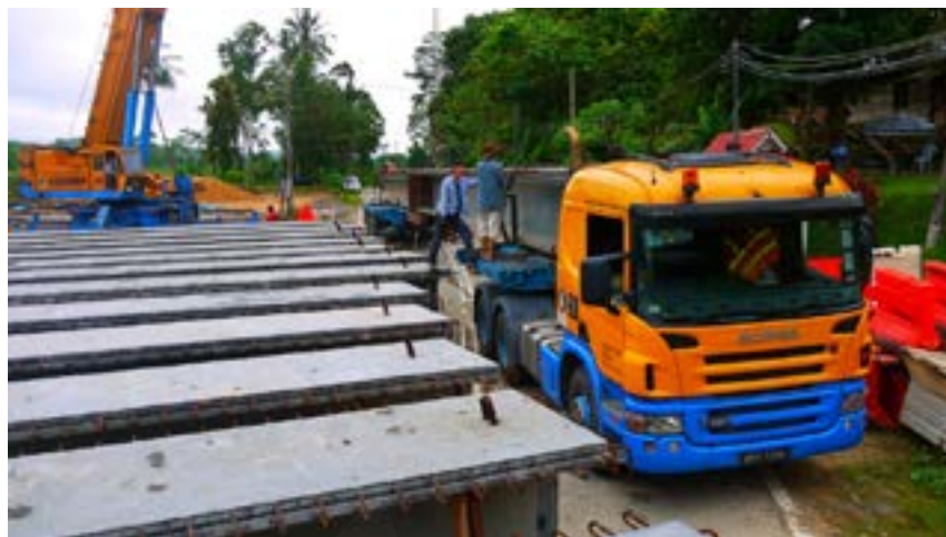
Fig. 5-187 Girder arriving at bridge construction site, where it will be placed in temporary storage until needed for installation.
