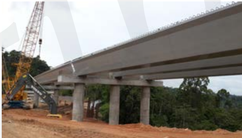
Fig. 5-203 Preparing to form a diaphragm on a pier beam on this bridge, similar to the example.
