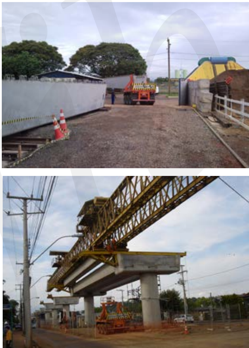
Fig. 5-62 Examples of transporting and installing girders.
