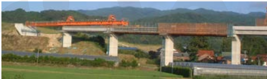
Fig. 5-143 Erection using an erection girder.
