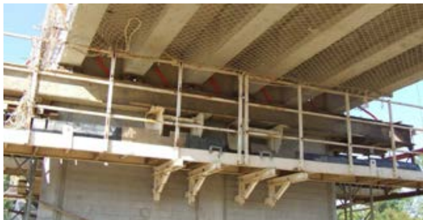
Fig. 5-98 Example of temporary support fastened to the pier.
