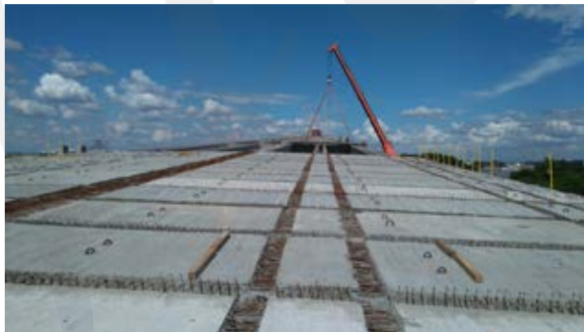
Fig. 5-68 Typical precast concrete panel installation.
