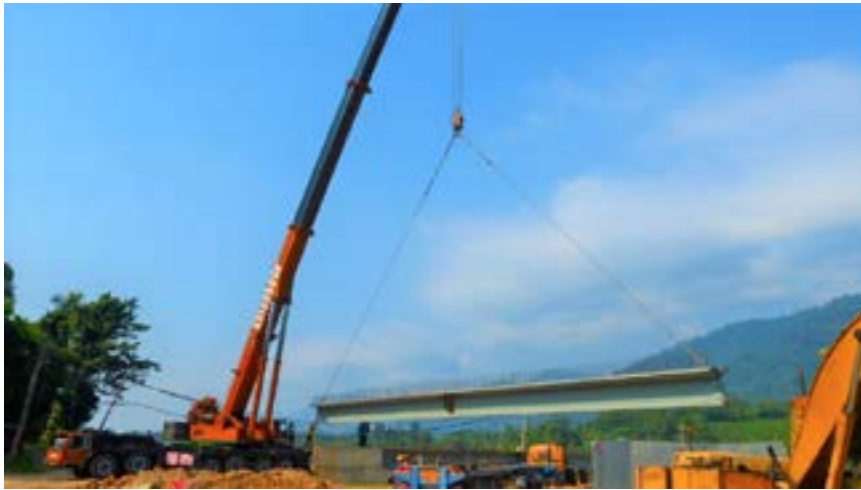
Fig. 5-189 The decked T girders are light enough to permit lifting by a single crane.
