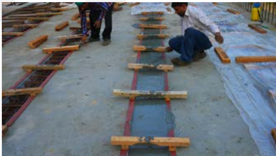
Fig. 5-194 Final hand-finishing of the joint.
