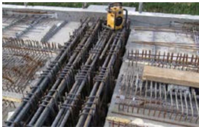
Fig. 5-26 Typical diaphragm reinforcement at a pier.
