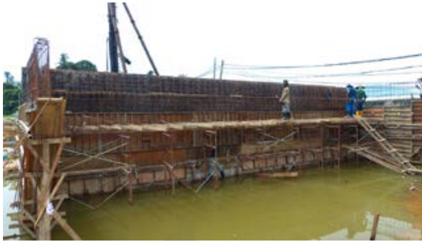
Fig. 5-184 Example of construction of an abutment shown from the approach side.
