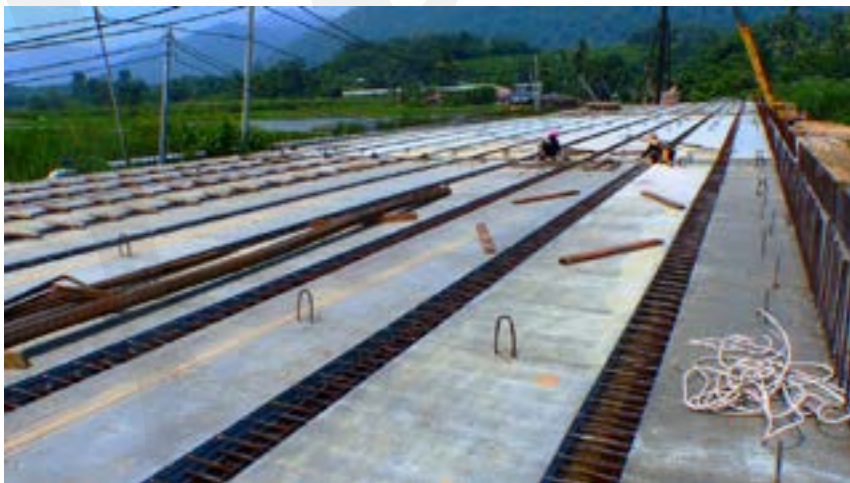
Fig. 5-191 The 300 mm (12 in.) wide spaces will be filled with ultra-high-performance fiber-reinforced concrete and will develop the bars in that distance.
