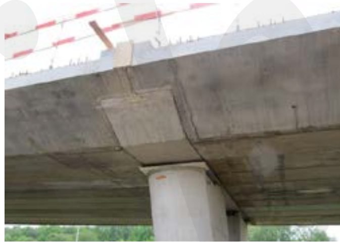
Fig. 5-21 Photo of the precast concrete pier beam at the edge of the bridge.
