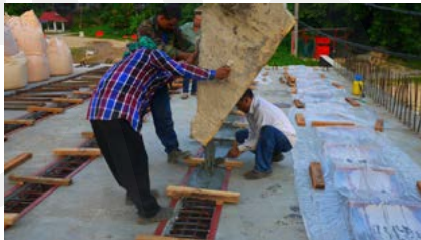
Fig. 5-193 Ultra-high-strength fiber-reinforced concrete being placed using a tremie, then leveled.
