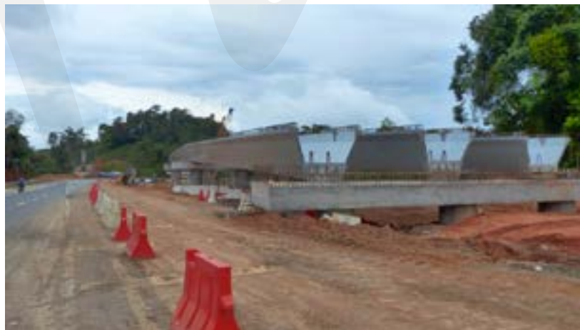
c) Construction of similar bridge nearly ready for forming the diaphragm
