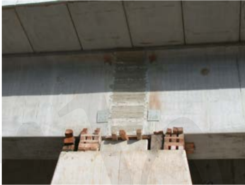
Fig. 5-112 Example of full continuity in the “Quattro Querce” Viaduct .
