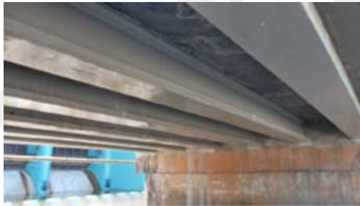
Fig. 5-162 Connection over piers.
