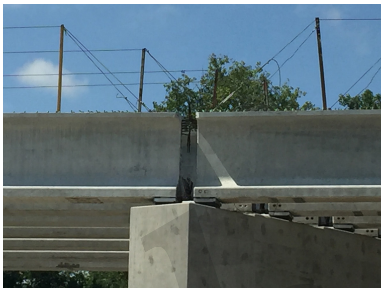
Fig. 9-5 Bridge under construction near Des Moines, Iowa, US. Note bent strands
