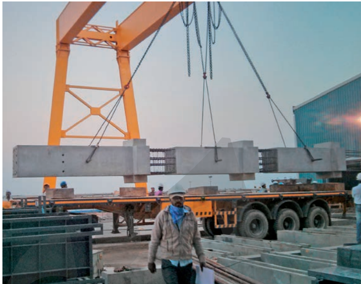
Fig. 5-47 Lifting of column with two gaps after demoulding for transport, Cummins project, Pune, India (Credit for above photos - Nagesh Kole; photos courtesy of Precast India Infrastructures Pvt. Ltd)
