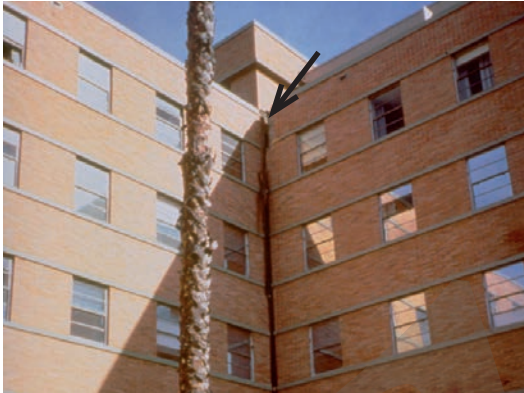
Fig. 3-19 Damage to hospital building in Sepulveda (USA) after 1994 earthquake. Seismic joints separated and blocks pounded together (Photo courtesy of NOAA/NGDC, Mehmet Celebi, US Geological Survey)
