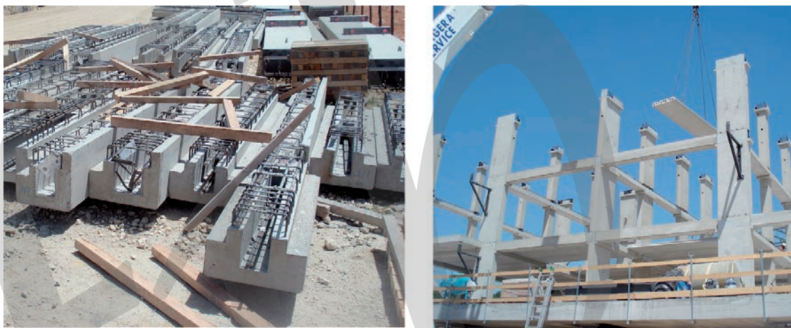
Fig. 5-34 Application of System S2 in Italy Left: Shell beams are supported in small column corbels Right: Slabs seated in beam ledges (C.A.S.E. project - L' Aquila earthquake - April 6, 2009; photos courtesy of Stefano Pampanin)
