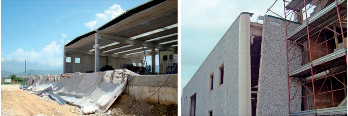
Fig. 3-27 Out-of-plane collapse of cladding panels during L'Aquila earthquake, 2009 (Toniolo and Colombo, 2012)
