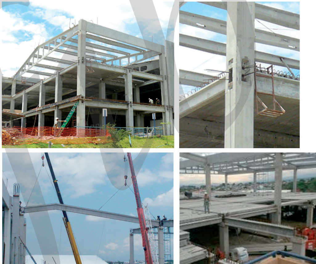
Fig. 5-67 Practical application of post-tensioned jointed ductile connections for two- and three-story industrial buildings in Costa Rica (Photos courtesy of Productos de Concreto S.A.)
