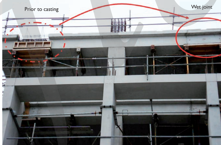
Fig. 5-36 Application of emulative approach using System S3 in IRD Building, Christchurch, New Zealand (Photo courtesy of Stefano Pampanin)
