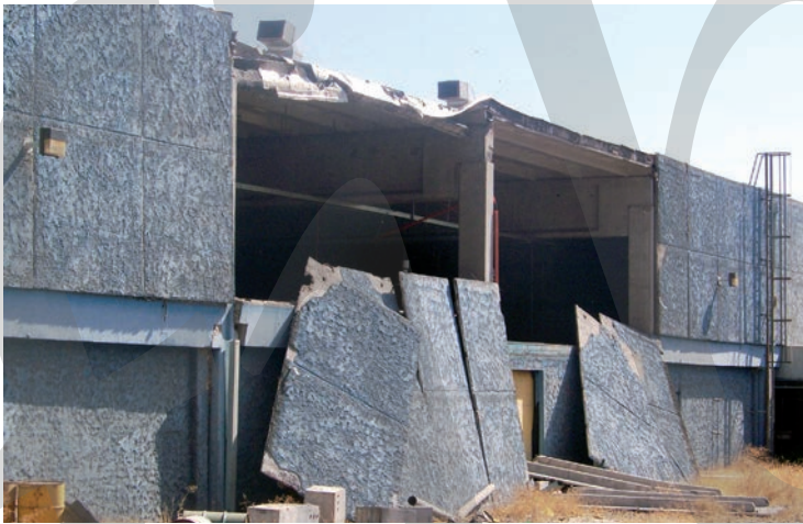
Fig. 3-28 Collapse of panels during Chile earthquake, 2010
