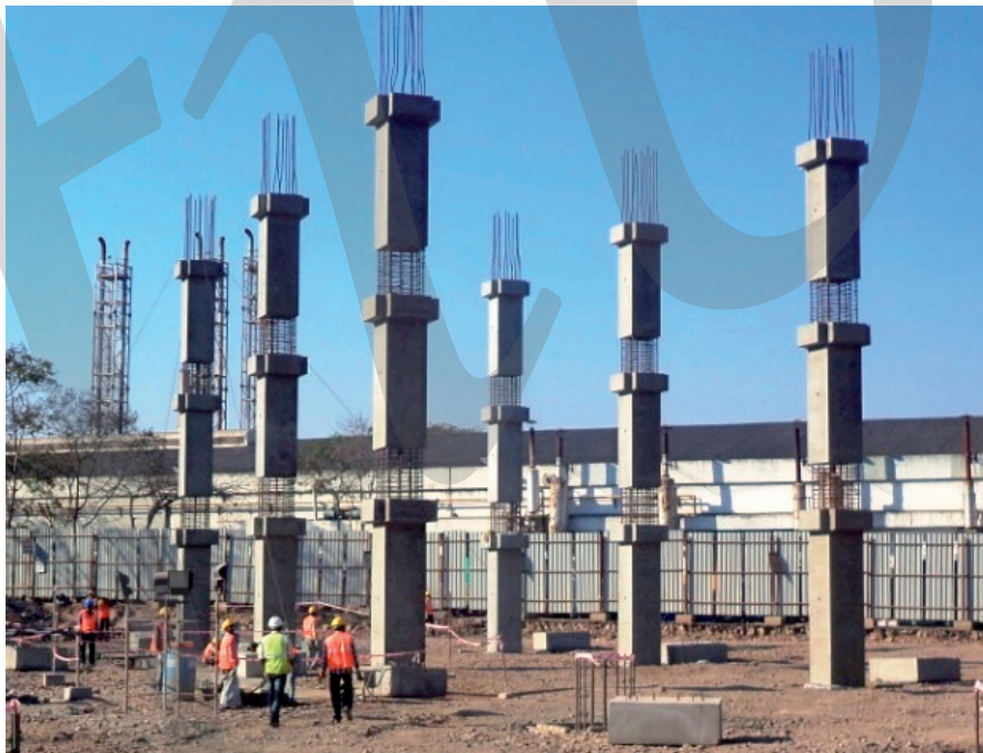
Fig. 5-46 Cummins precast project (Cummins) in Pune, India, implementing System S7 (photo credit - Nagesh Kole; photo courtesy of Precast India Infrastructures Pvt. Ltd)
