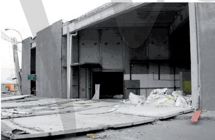
Fig. 3-29 Collapsed panel due to connection failure at roof level, Chile, 2010
