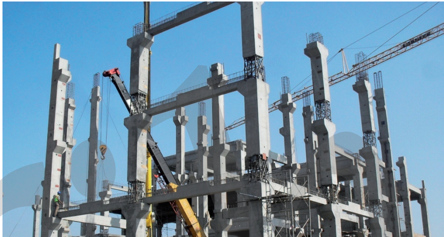
Fig. 5-45 Schmersal precast project in Pune, India, implementing System S7 (photo credit - Nagesh Kole; photo courtesy of Precast India Infrastructures Pvt. Ltd)
