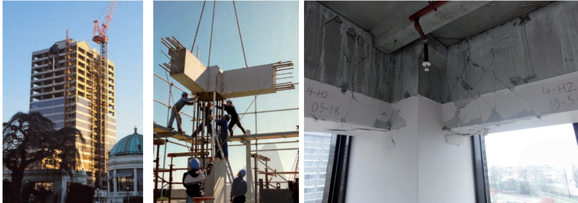
Fig. 5-53 Beam plastic hinges in a mid-1980s 22-story reinforced-concrete building based on System 2 and demolished after the Canterbury earthquakes of 2010 to 2011 Left and centre: Building under construction (photos courtesy of J. Restrepo) Right: Damage to plastic hinge after 22 February 2011 quake and aftershocks and prior to demolition (photo courtesy of S. Pampanin)
