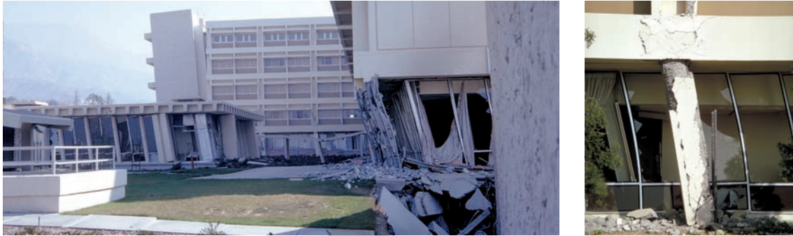
Fig. 3-23 Olive View Hospital, San Fernando earthquake, 1971, showing extreme deformation of columns above plaza level (Photos courtesy of NISEE-PEER, University of California, Berkeley)
