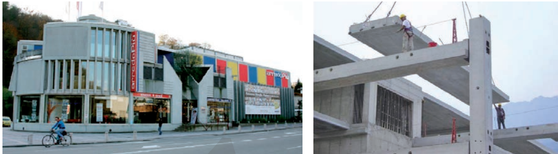
Fig. 5-58 Rendering and application of post-tensioned solution with draped tendons, particular to Brooklyn System, developed by BS Italia, Bergamo, Italy (Pampanin et al., 2004)
