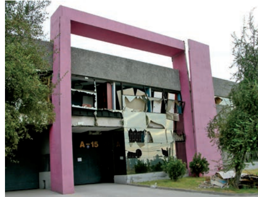
Fig. 3-31 Damaged precast-concrete cladding, Chile 2010 (Ghosh and Cleland, 2012)
