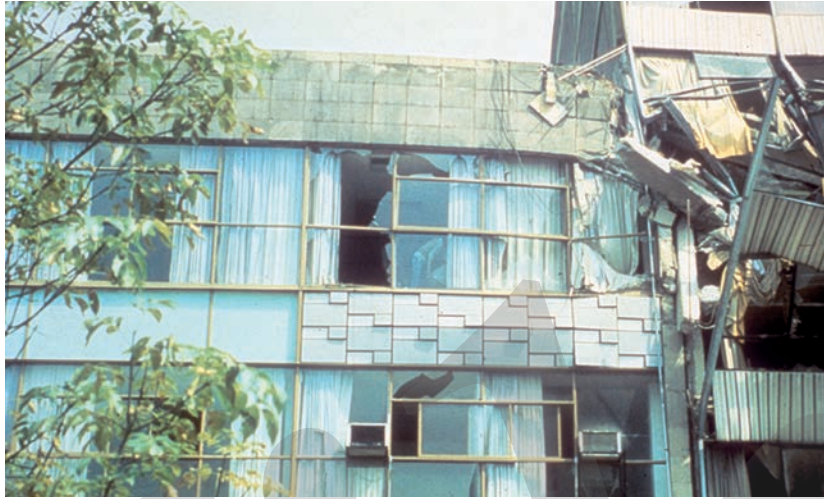
Fig. 3-16 Detail of damage to Hotel de Carlo, showing intermediate floor failure (Photo courtesy of NISEE-PEER, University of California, Berkeley)
