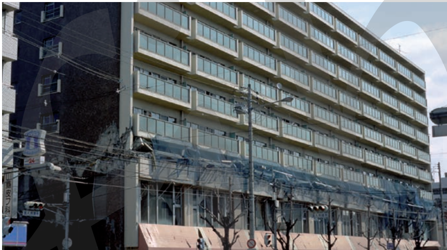
Fig. 3-24 Soft-storey or 'pancake' collapse of the third floor of a building during Kobe earthquake, Japan, 1995 (Photo courtesy of NISEE-PEER, University of California, Berkeley)
