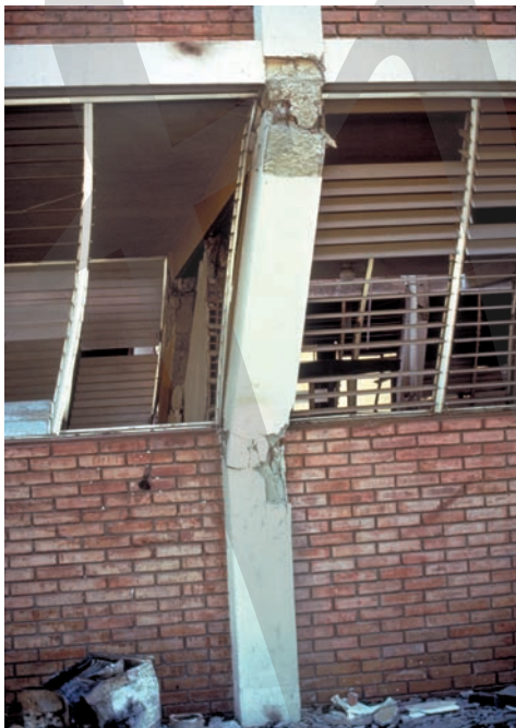
Fig. 3-26 Shear failure of columns under shear forces induced by inadequate arrangement of infills
