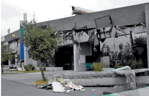
Fig. 3-30 Precast-concrete cladding collapsed as supporting structure underwent local failure, Chile 2010 (Ghosh and Cleland, 2012)
