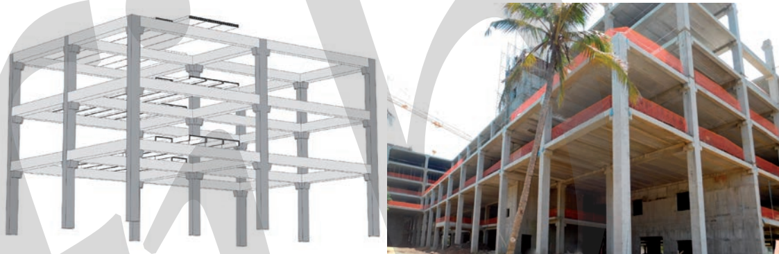
Fig. 5-2 Left: Typical HCF structural system (hinged beam-to-column connections and fixed column-to-foundation connections) Right: Case under construction in Calicut, Kerala, India (Photo credit: A Dienst; photo provided courtesy of KEF Infrastructure India Pvt. Ltd)
