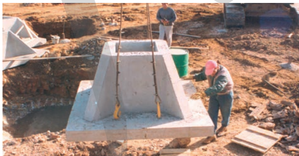
Fig. 5-69 Typical socket foundation with side starter bars for connection with tie-beams: a. before concreting the foundation base; b. after concreting the foundation base (Photos courtesy of ASPROKAT S.A., Aspropyrgos, Greece)
