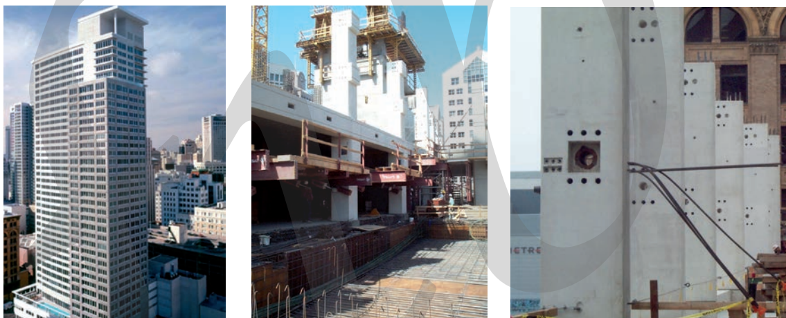
Fig. 5-63 Left: Completed Paramount Building, San Francisco, California Centre and right: On-site applications of unbonded post-tensioned hybrid frames in Paramount Building (Photos courtesy of Charles Pankow Builders, Ltd.)
