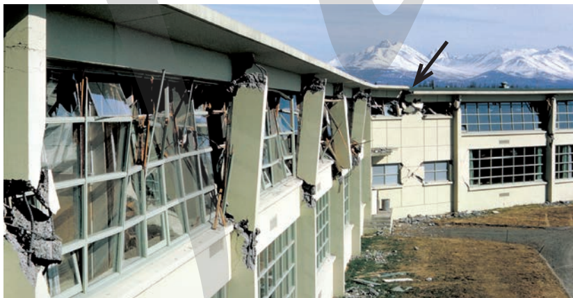
Fig. 3-18 Damage due to stress concentration at notch of shallow L shaped building (West Anchorage High School) after 1964 Alaska earthquake (Photo courtesy of NISEE-PEER, University of California, Berkeley)
