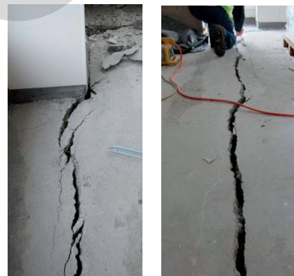
Fig. 8-4 Extensive damage to floor diaphragm and loss of floor support in ductile RC multi-storey frame building caused by beam-elongation effect during Christchurch earthquake of 22 February 2011 (Pampanin et al., 2012; Kam et al., 2011)
