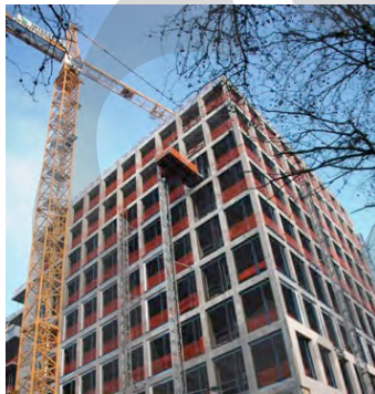
Fig. 4.6: Building structure with Pi-elements and HC floors in Brussels, Belgium
