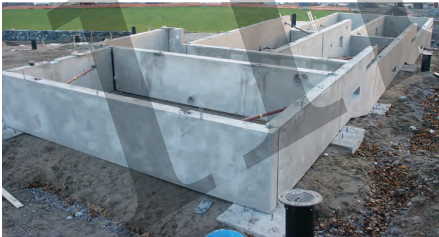
Fig. 7.27: Foundation walls for single-family housing
