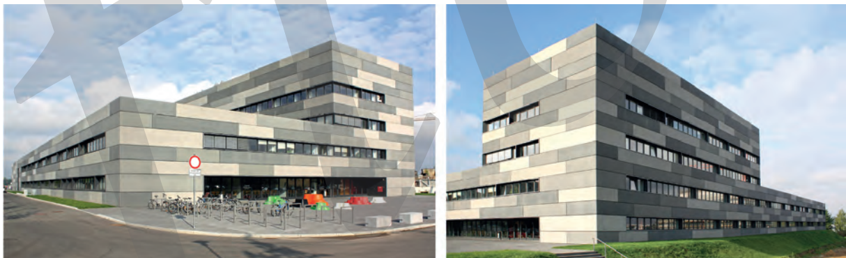
Fig. 1.26: White cement and dark granite gravel were used for the façade panels of the Institute of Physics at the Chemnitz University of Technology, Germany
