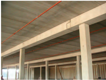
Fig. 6.38: Reinforced concrete inverted-tee beams designed with a scarf joint at approximately 750 mm from the face of the column creates a negative bending moment at the column that will reduce the depth of the beam
