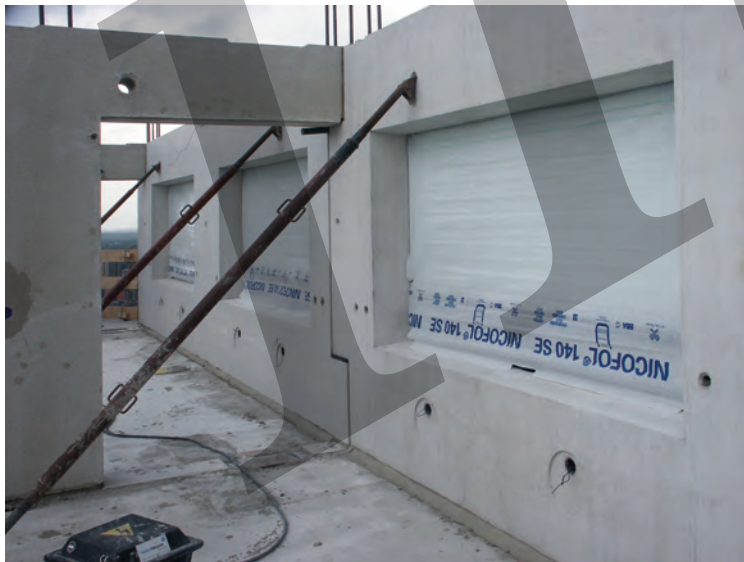
Fig. 5.16: Transfer of shear forces by staggered joints in wall panels
