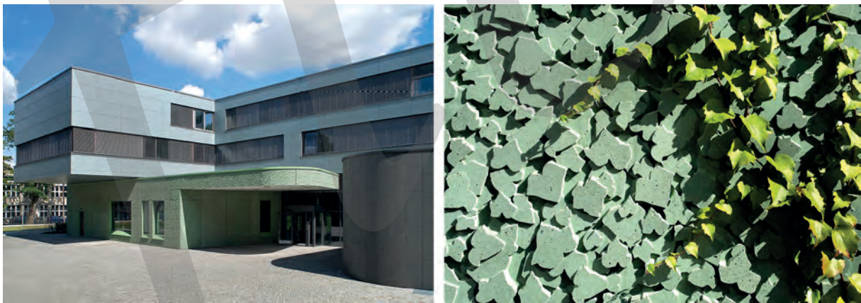
Fig. 1.22: The façade panels were produced using silicone moulds
