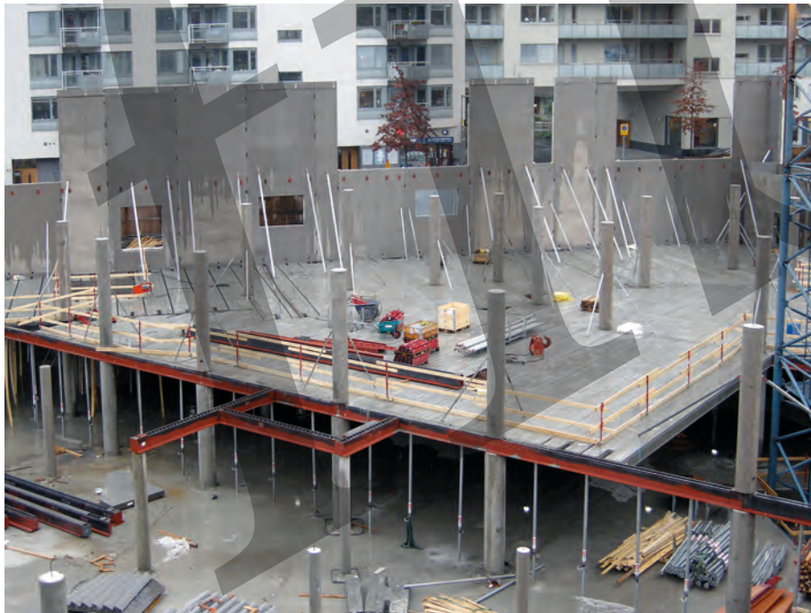
Fig. 8.32: Hollow-core floor supported on hat beams
