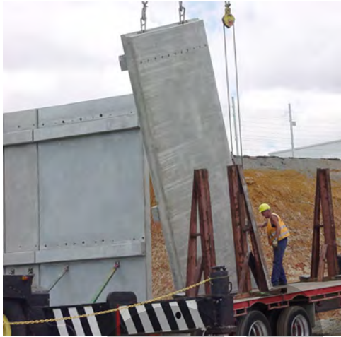
Fig. 7.26: Application example of two-storey height precast retaining walls
