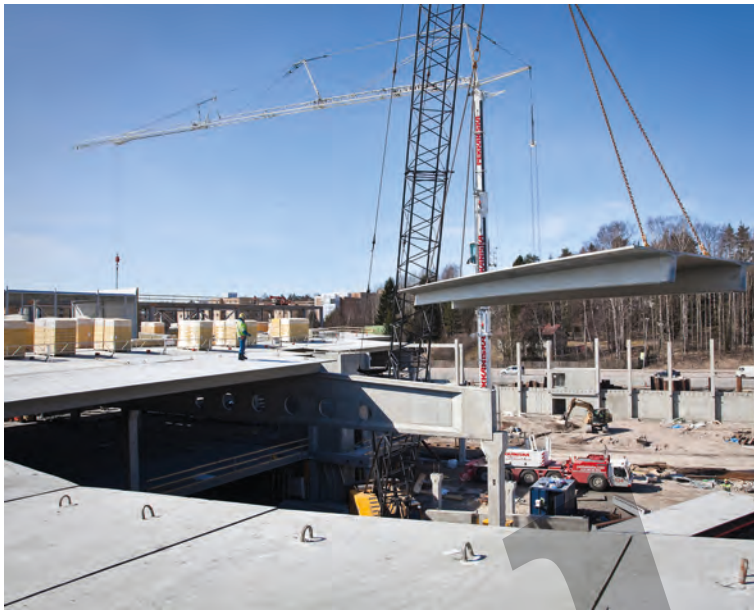
Fig. 8.7: Ribbed roof elements for an industrial hall
