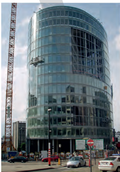
Fig. 1.3: Flexibility in design and construction enables this oval shape building in Brussels, Belgium, to be prefabricated with mainly rectangular concrete elements
