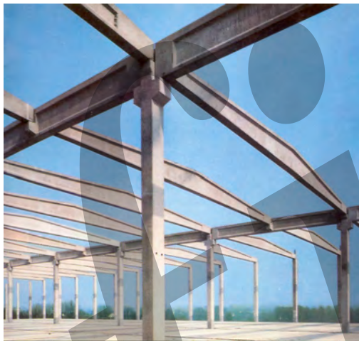
Fig. 6.56: Beam-to-beam connection using a corbel at mid span of the primary roof beam
