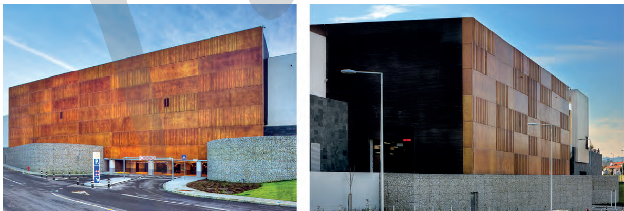
Fig. 1.18: Shopping centre, Guimaraes, Portugal. The precast façade panels are finished with a special technique to give them the appearance of weathered corten steel.
