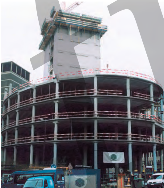
Fig. 6.17: Precast concrete skeletal frame braced against horizontal forces by in-situ core
