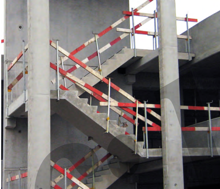
Fig. 7.32: Application example of stair and flight connections with corbels and beams
