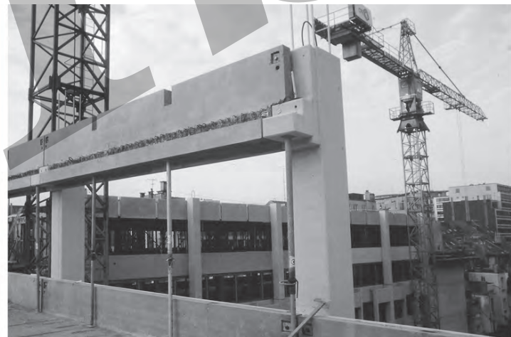
Fig. 6.14: Skeletal framework with load-bearing spandrel beams
