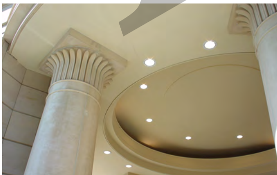
Fig. 9.9: Reconstructed stone precast concrete columns for entrance of apartment building
