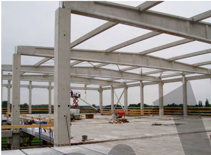
Fig. 6.33: Portal structure with roof rafters and purlins
