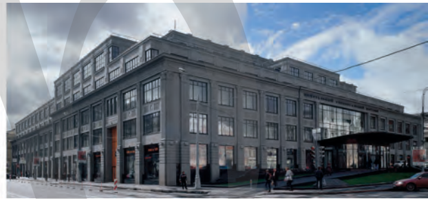
Renovated façade of the TsUM shopping centre in Moscow. The precast façade units were manufactured in Belgium and transported over a distance of more than 3500 km.
