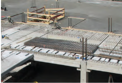
Fig. 6.23: Prestressed hollow-core floor units prepared for the additional structural topping, giving a total depth of 260 mm or a span/depth ratio equal to 35
