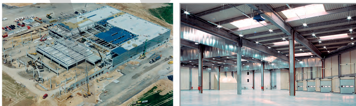
Fig. 1.33: Industrial buildings in Belgium, with a portal frame consisting of rigid founded columns and simply supported rafters
