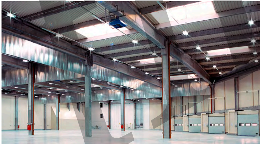
Fig. 6.1: Portal frame consisting of rigidly founded columns and simply supported rafters
