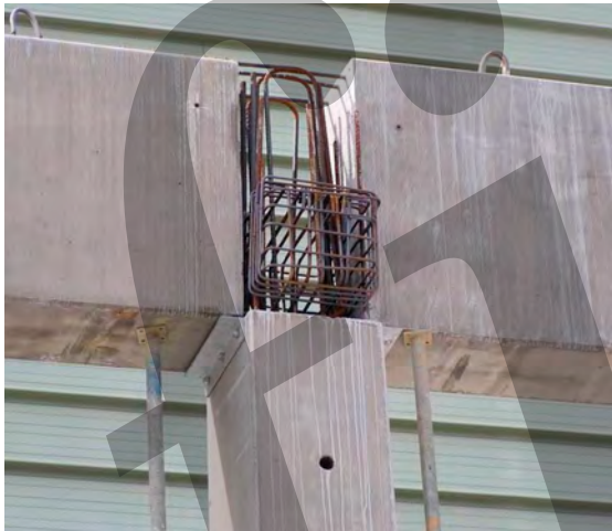
Fig. 5.31: Example of an extended bearing
