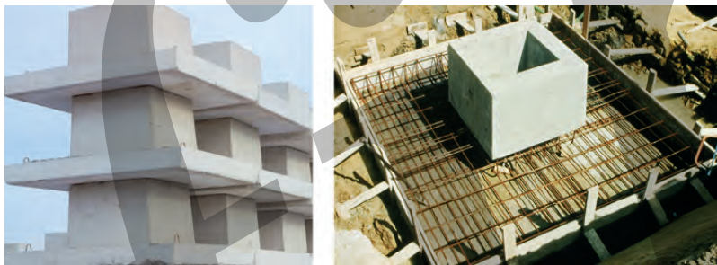
Fig. 6.42: Precast pocket foundations are an alternative to site cast pockets, particularly if the foundations cannot be prepared in time for the installation of the column Left: Totally precast Right: Precast pocket and cast-in-situ slab
