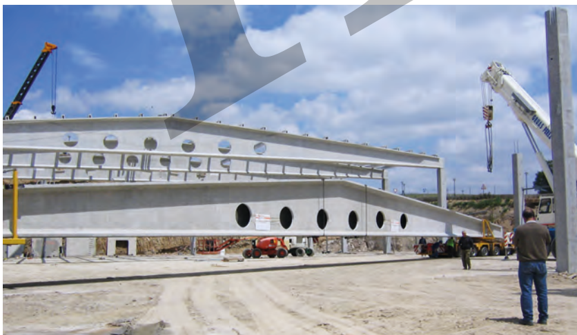
Fig. 6.6: Erection of 52m-long roof rafters with two mobile cranes for a project in Salamanca, Spain
