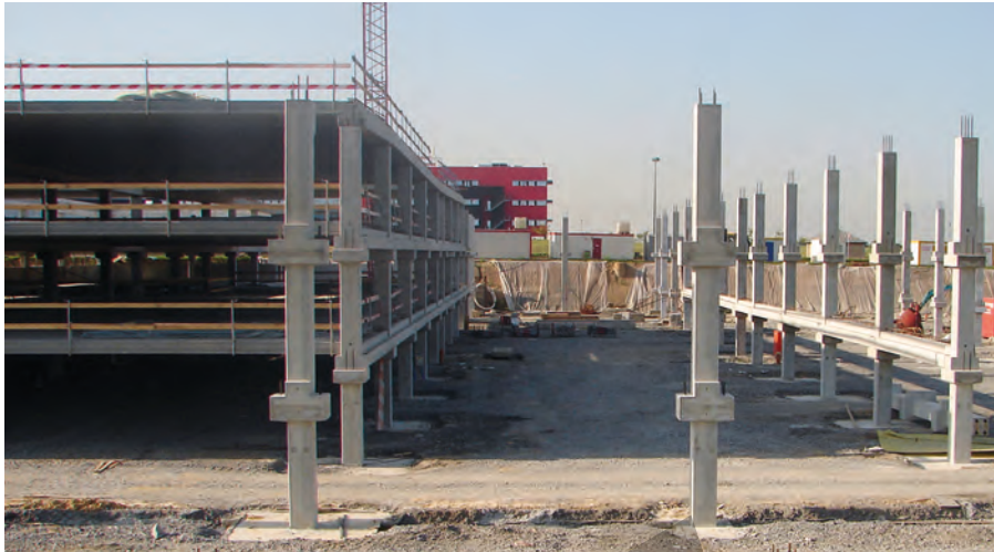
Fig. 6.25: Precast concrete skeletal frame for car park, designed using the columns acting as vertical cantilevers to resist horizontal forces and drift
