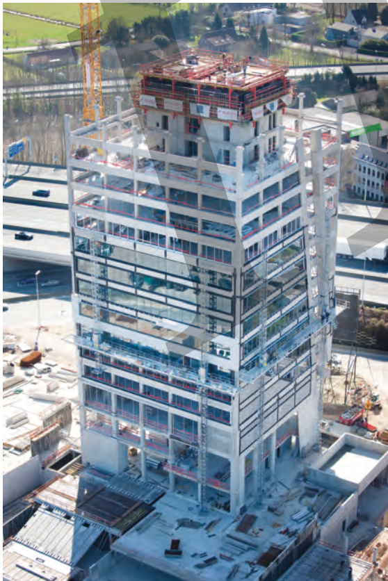
Fig. 6.26: Precast skeletal structure braced by a cast-in-situ central core
