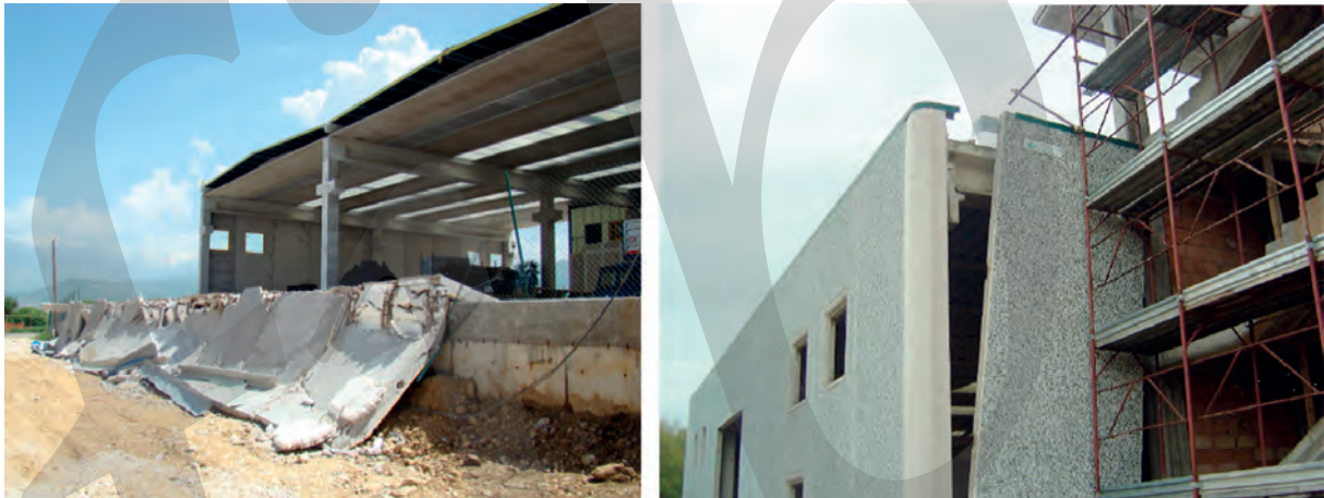
Fig. 2.14: Out-of-plane collapse of cladding panels during the L'Aquila earthquake, 2009 [49], due to inadequate connections of cladding to the bearing members
