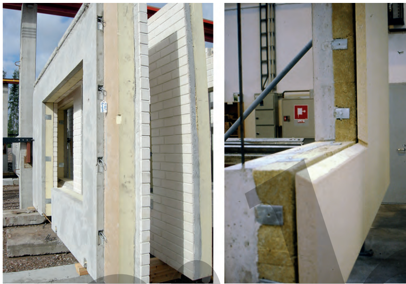
Fig. 9.6: Sandwich panels
