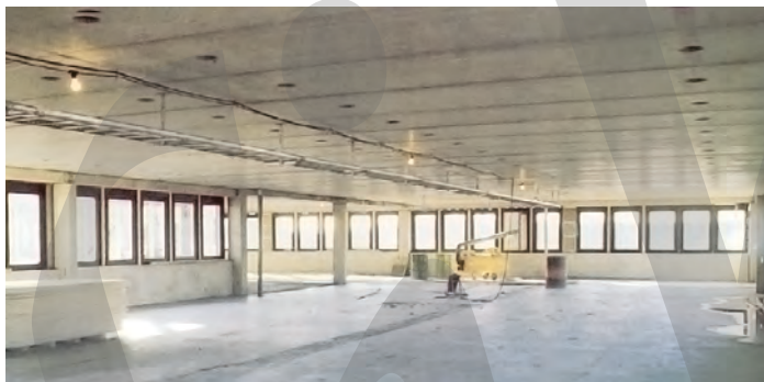
Fig. 3.14: Modern office building with hollow core floors spanning from one façade to the other
