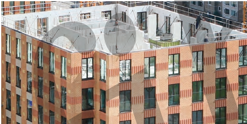
Fig. 7.9: Precast core with single-storey panels, connected by a combination of wet-shear joints for a project in the Netherlands
