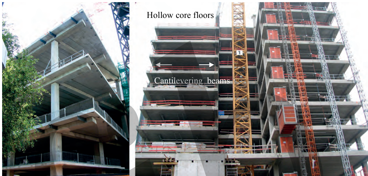
Fig. 8.22: Examples of precast cantilevering beams over columns
