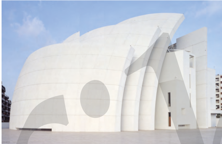
Fig. 1.34: The Jubilee Church in Rome, where the 'sails' are composed of double-curvature precast panels in white concrete with marble aggregate, assembled by post-tensioning
