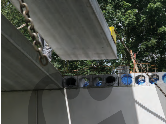
Fig. 5.60: Typical floor-wall connection without wall corbels
