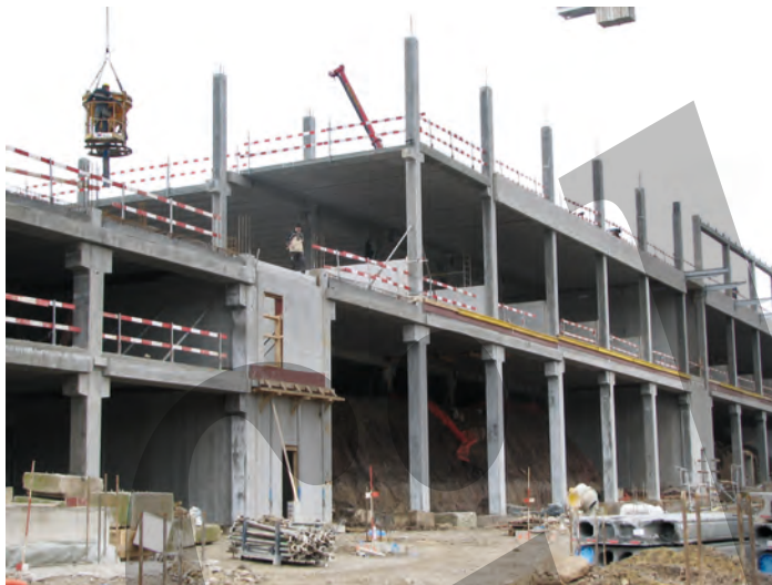
Fig. 6.2: Precast concrete skeletal frame, designed as a braced structure using precast shear walls with long-span prestressed concrete floors acting as a horizontal plate between them
