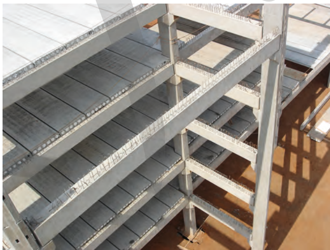
Fig. 2.2: Achieving simplicity of design and construction for beam connections (ABCIC Brazil)
