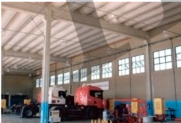
Fig. 6.32: Precast concrete portal with primary I-section beams and trough section roof units
