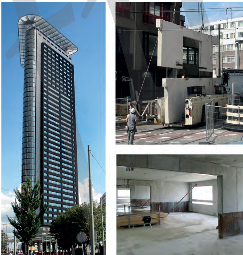
Fig. 4.9: Precast concrete shear walls used to brace a 45-storey wall-frame structure in Den Hague, The Netherlands. Storey-high shear-wall panels are connected in such a way that the whole building can function as a cantilevering tube.
