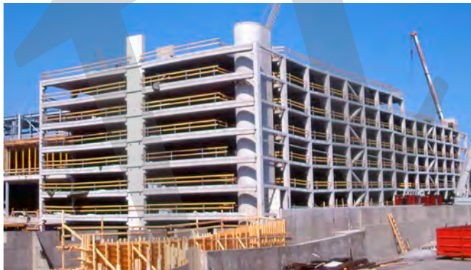
Fig. 4.4: Precast car park using three different bracing systems: deep columns (known as wind posts, left), stair core and diagonal strut and tie.
