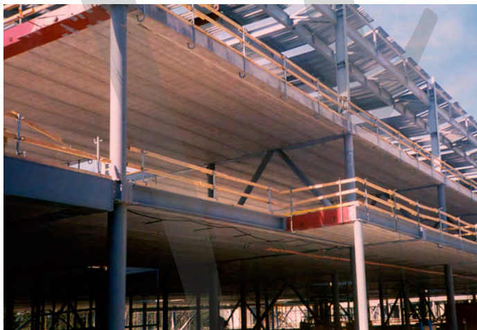
Fig. 2.21: Mixed steelwork and precast concrete at the Big Apple retail centre near Helsinki, Finland
