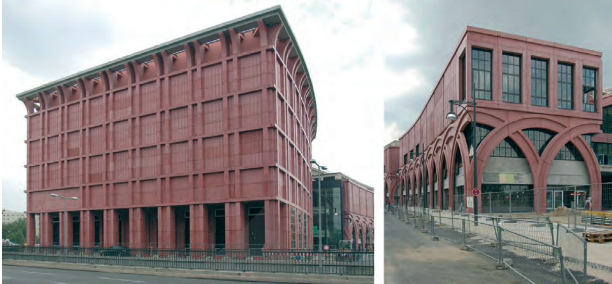
Fig. 1.29: Three-dimensional, CNC-supported formwork construction for the Alexa shopping centre in Berlin, Germany
