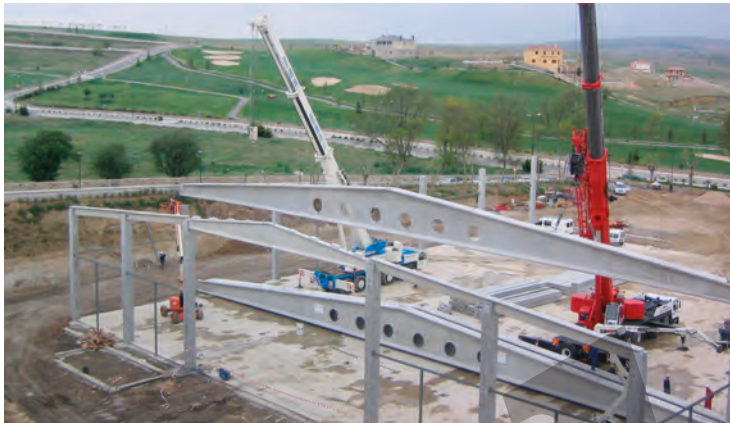
Fig. 6.4: Roof structure with rafters for the long span and T-shaped rectangular beams for the smaller spans, Salamanca, Spain
