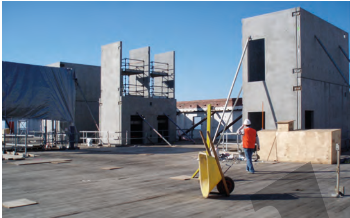
Fig. 7.8: Precast core with two-storey-high wall panels, connected temporarily during erection by bolting, followed by welding of cast-in anchor plates
