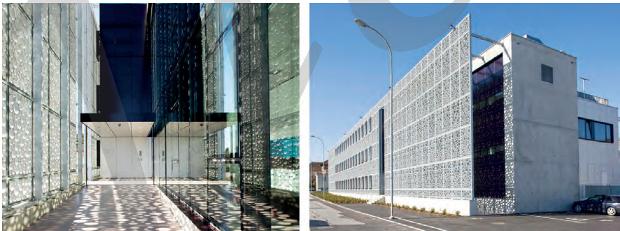
Fig. 1.15: A free-standing façade made of precast concrete elements serving as a sun filter, in Cormondrèche, Switzerland
