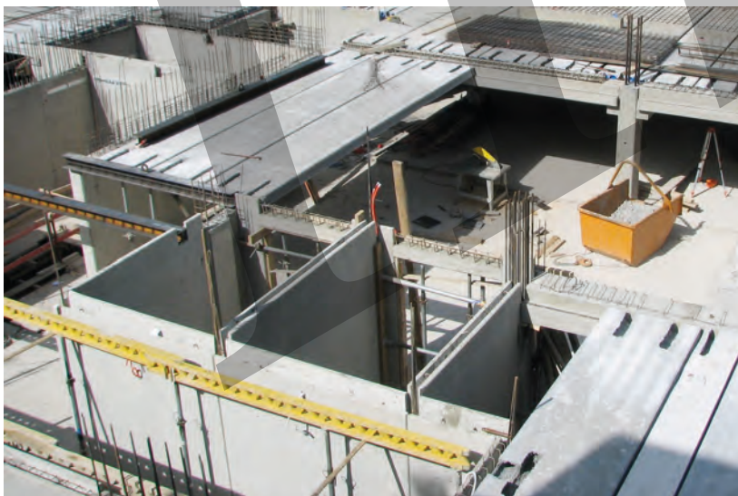
Fig. 7.25: Application example of twin wall system for a central core
