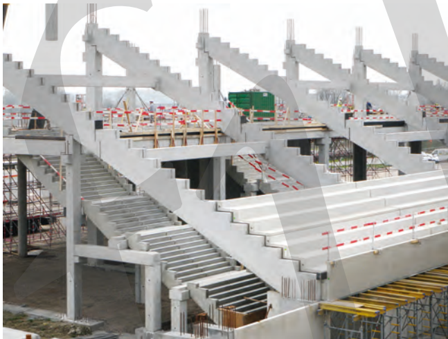
Fig. 3.22: Precast raker (inclined) beams support precast terraces at Ghelamco Arena, Ghent Belgium
