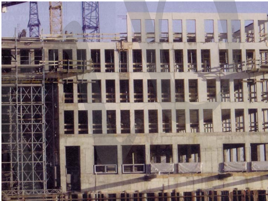
Fig. 9-1: Moment resisting perimeter frame (Courtesy BFT Journal)
