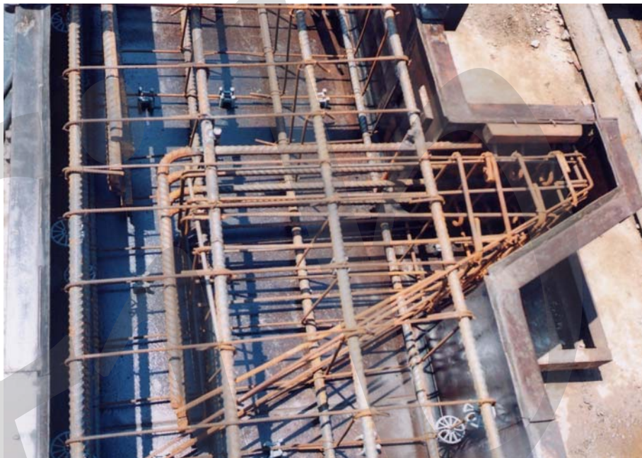
Fig. 9-18: Reinforcement arrangement for corbel
