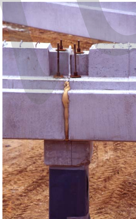
Fig. 9-27: Construction of beam-column head connection
