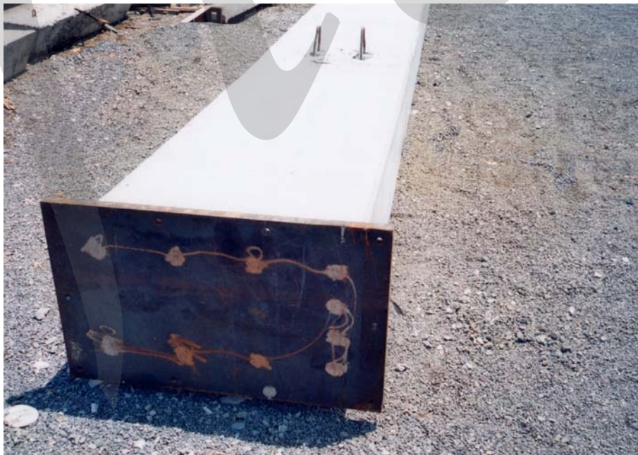
Fig. 9-40: Construction of steel base plate, showing starter bars are welded through holes in the plate
