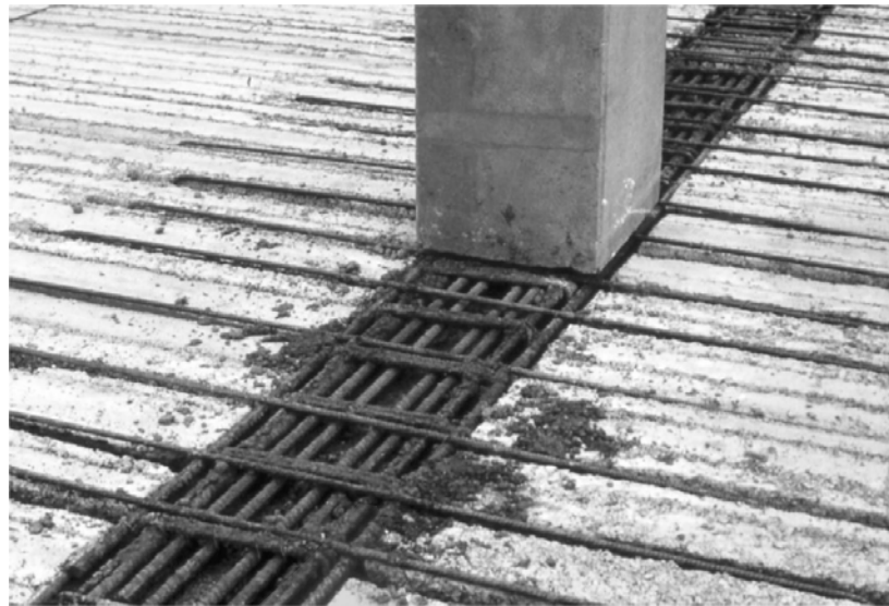
Fig. 9-43: Negative moment continuity reinforcement placed into top opened cores in precast hollow core units. Transverse reinforcement parallel with the beams also provides moment continuity through the column (Courtesy APE and GRUPPO CENTRO NORD)
