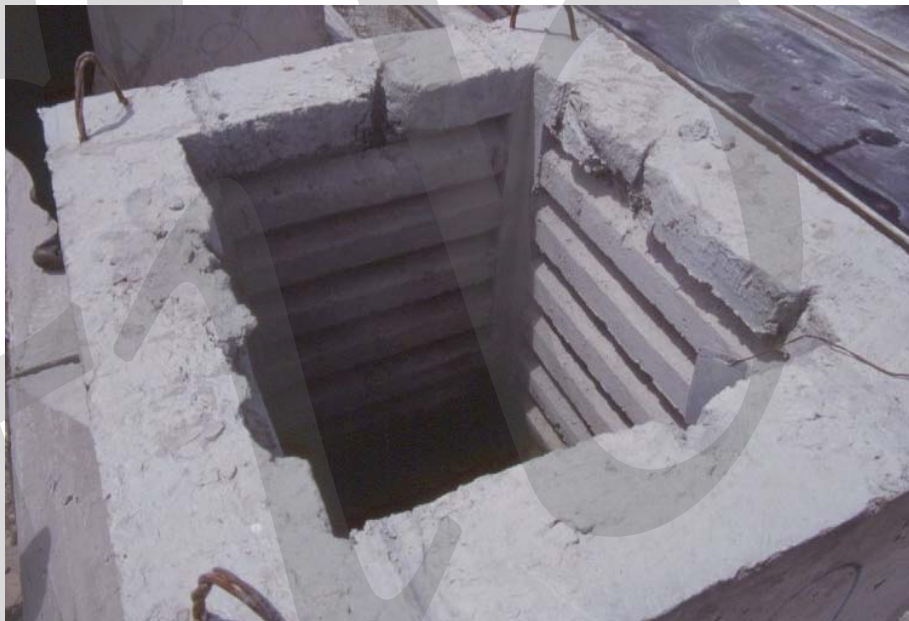
Fig. 9-36: Precast concrete column pocket foundations, with castellations for enhanced bond to the column
