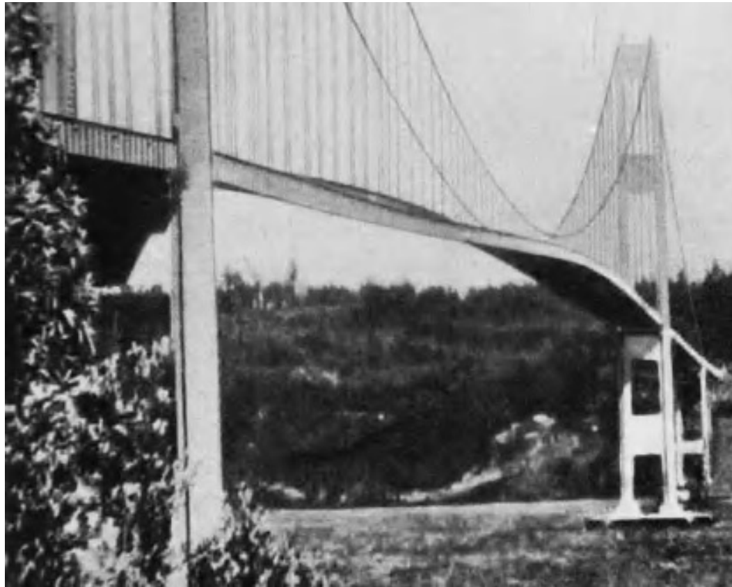
Tacoma Narrows Bridge shortly before collapse 1940
