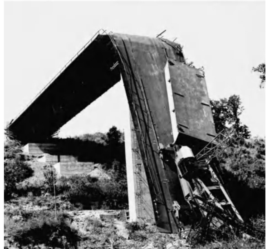
Zeulenroda reservoir Bridge, 1973-- after failure. [Scheer, 2010]
