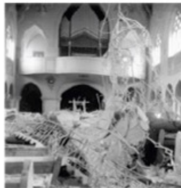
Figure 8: The 1946 earthquake of Sierre: Photographs of the collapsed ceiling in the church of Chippis and of the landslide off the Rawylhorn, triggered by an aftershock of the earthquake, as well as a map of the inferred macroseismic intensities.
