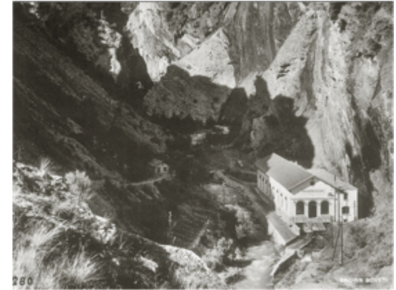
Hydropower station (Lonza) in Gampel 1897
