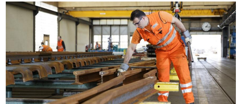
Refurbishment of rails : Reusing used rails when changing rails or in side tracks is also financially worthwhile.
