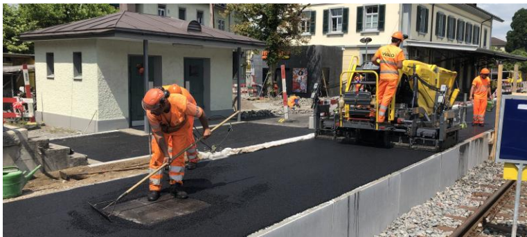
Standards adapted to recycled asphalt for platform construction. Reduce environmental impact by a quarter, business case neutral.
