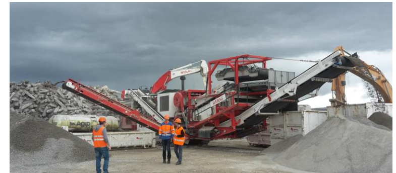
Breaking "old" SBB concrete sleepers with 40% recycled concrete content in new production. Improved environmental balance and resource conservation.
