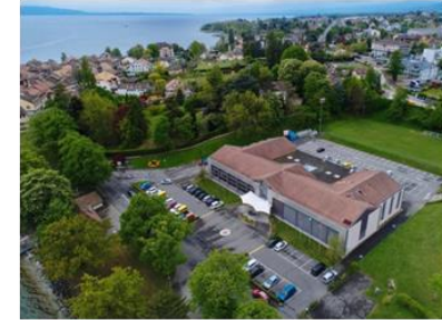
3 Energy renovation of Vieux Moulin
