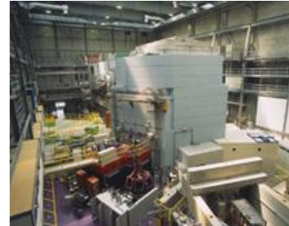
SINQ Spallation Source at PSI
