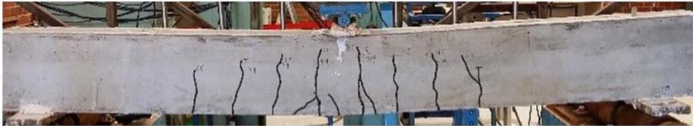
Failure under static load
