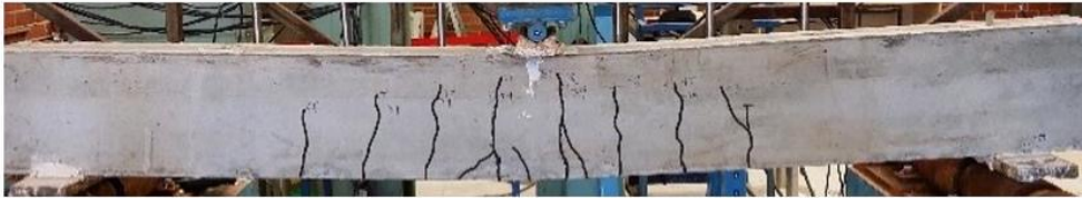
Failure under static load
