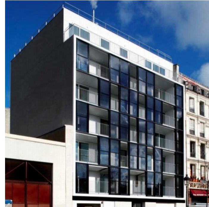
Glazed flat plate collectors integrated in building, Architect Philippon
