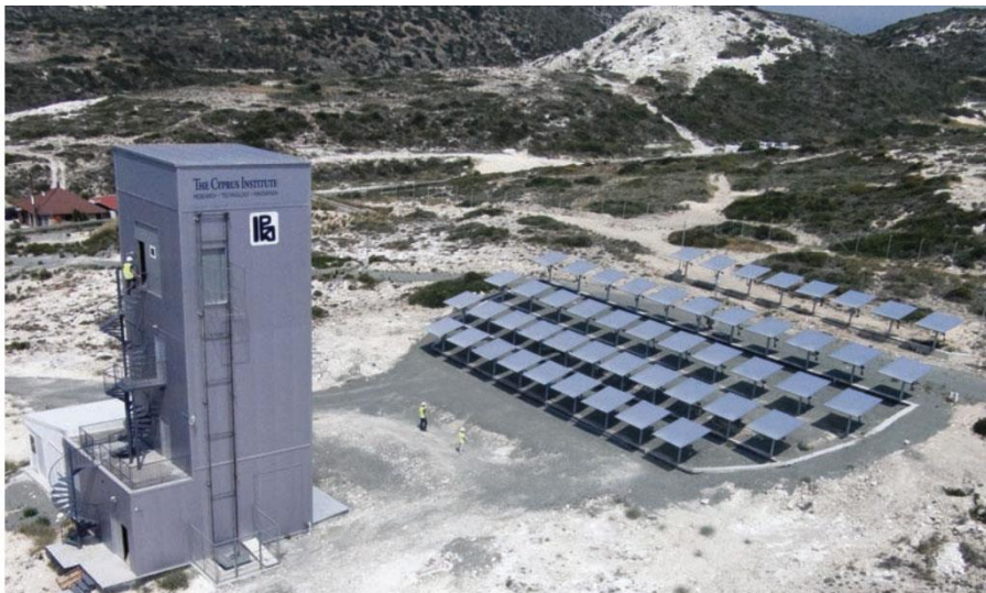
Pentakomo Field Facility: The rotating heliostats collect the light of the sun as it moves across the sky and redirect it onto a receiver on the top of the tower
