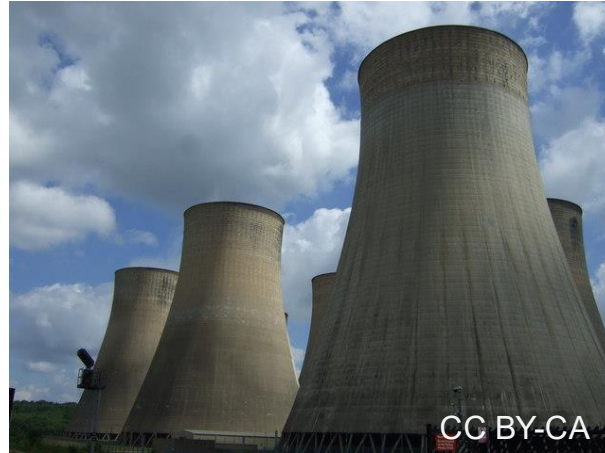
(nuclear) power plant
