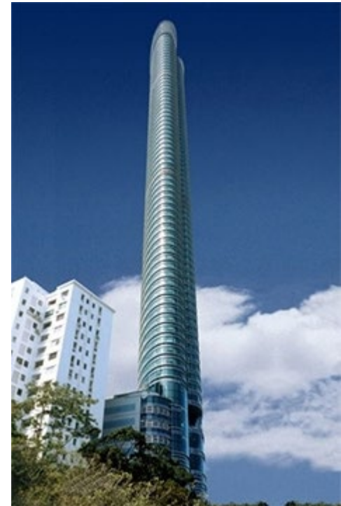
Tuned liquid “sloshing” mass damper Highcliff Apartments, Hong Kong, 1995.
