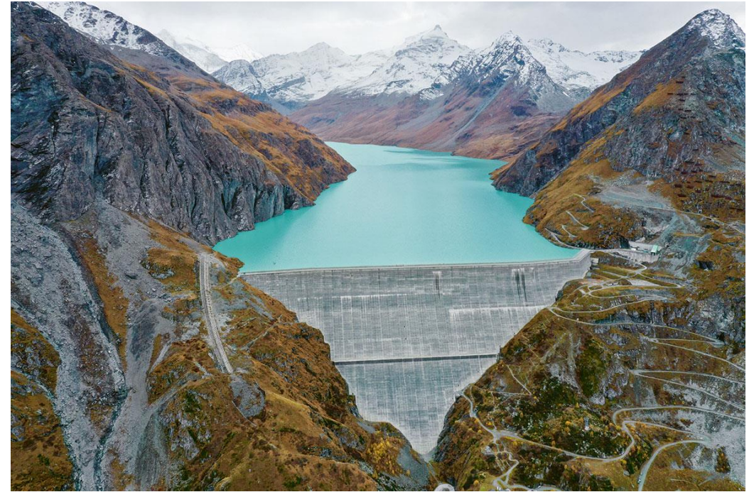
Credit: Jérémy Toma, CC BY-SA 4.0 Hydroelectric dam in Valais
