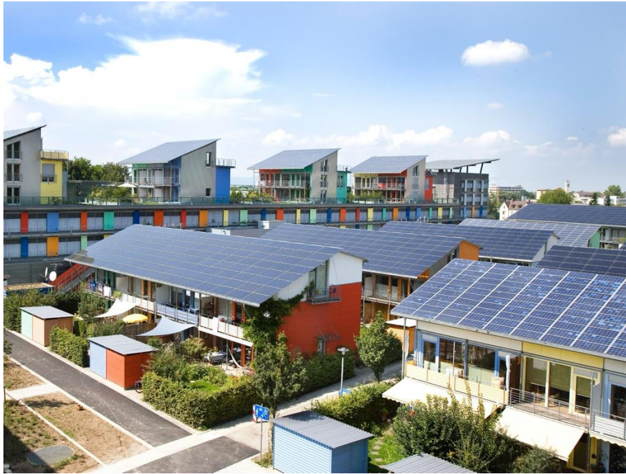
Credit: Andrewglaser, CC BY-SA 3.0 Solar photovoltaic panels
