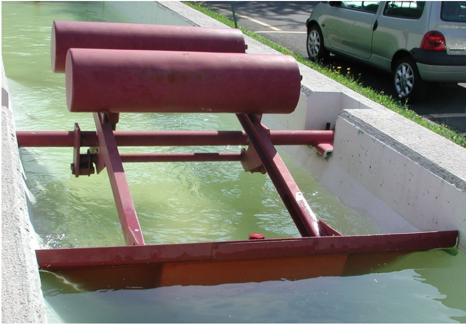
EPFL campus (irrigation loop)
