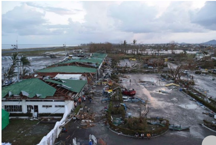
Tacloban airport damaged by Yolanda (Photo credits: sunstar.com.ph)
