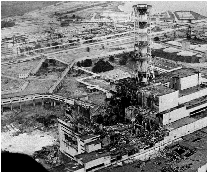
View of the reactor No 4 after explosion
