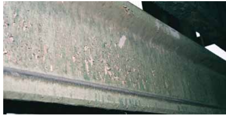
Fig. 4: Photo of girders taken during the inspection in 2000, showing scaled deposits and no visible corrosion
