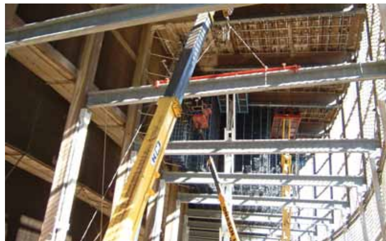
Fig. 1: Installation of the UHPFRC beams in 1997
