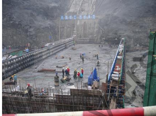
Fig. 5.8 - Preparation for concrete placement in Xiluodu Dam, China
