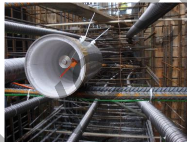
c) detail of "no-stress" strain enclosure
