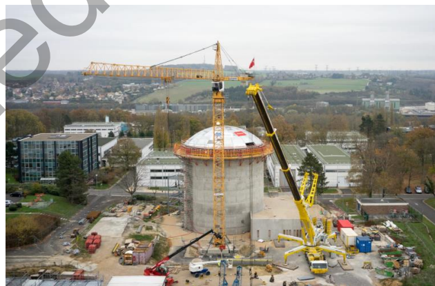
Fig. 9.34. VeRCoRS mock-up of a reactor containment building (Corbin and Garcia, 2016).
