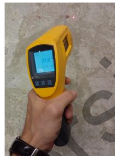
b) Surface temperature measurement of a concrete slab with infrared thermometer (photo: F. Kanavaris)
