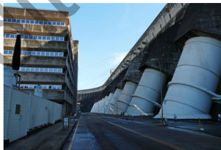
b) View of the intake
