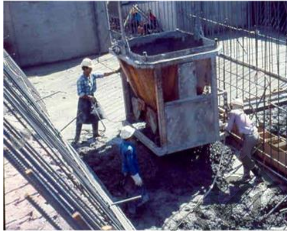
Fig. 5.10 - Placing stiff consistency concrete in Yacyretá Dam (Argentina - Paraguay)
