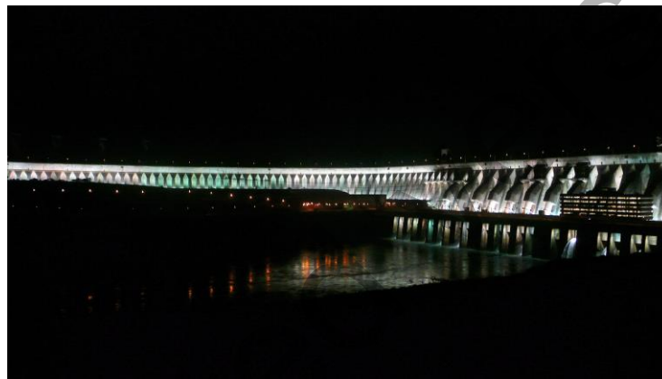
a) General view of the concrete dam
