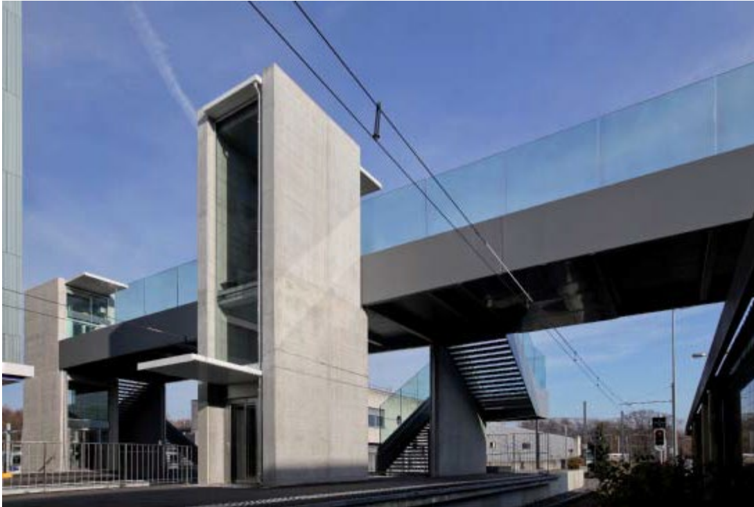
Figure 1: EPFL footbridge over M1 tracks, photo from Willi SA.
