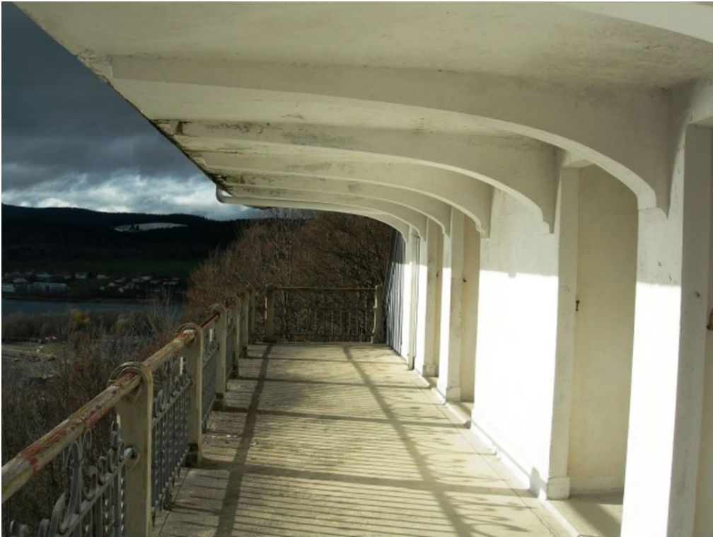
Figure 6: condition of the building in 2013, photo E. Brühwiler.
