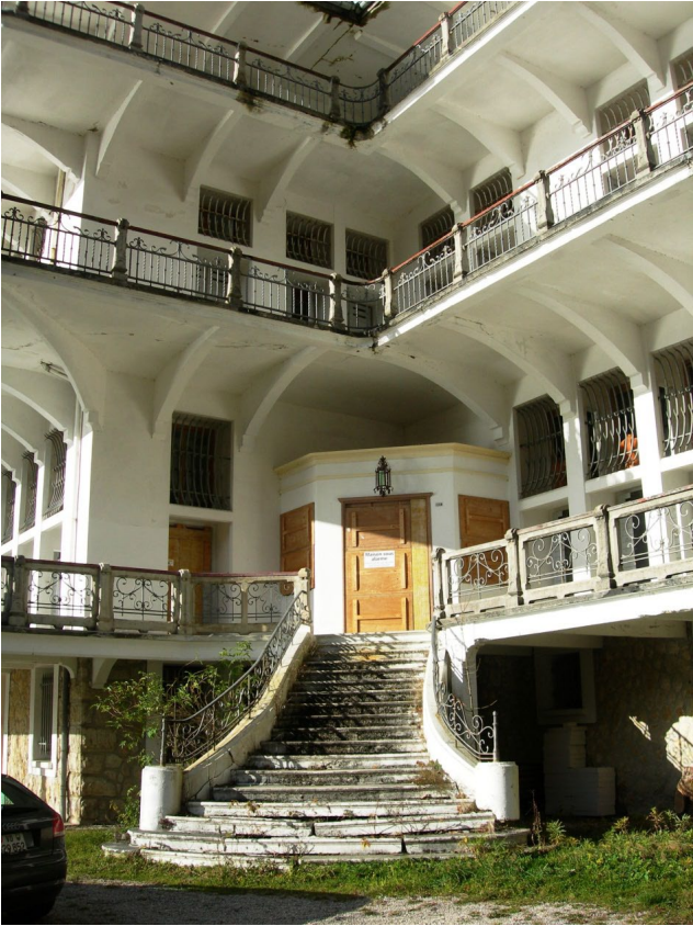
Figure 7: condition of the building in 2013, photo E. Brühwiler.
