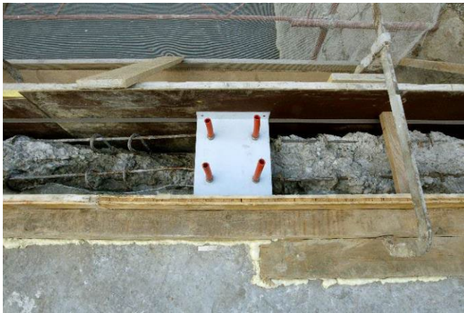
Existing kerb after hydrojetting
